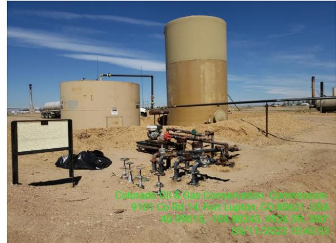
**Photo 9 Unused flow line has been removed .**
