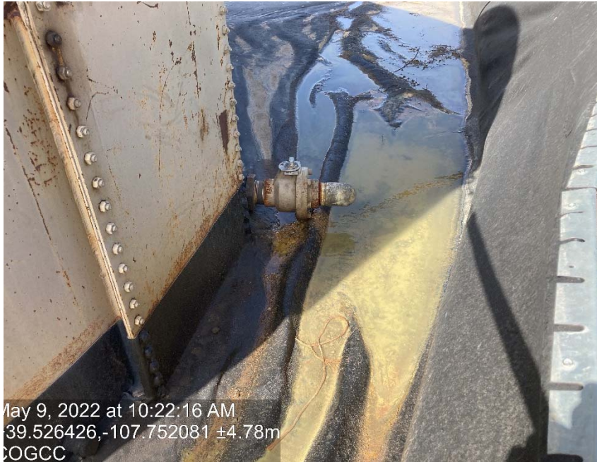
Valve on tank actively leaking
