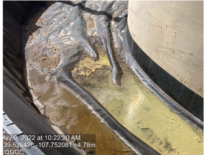
Valve on tank actively leaking
