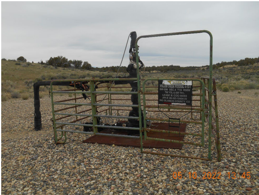
Injection wellhead
