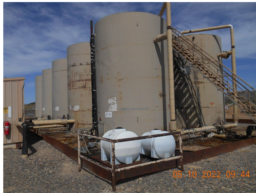
Tank battery offload station
