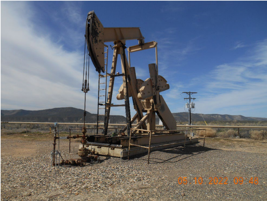
Pump jack on producing well
