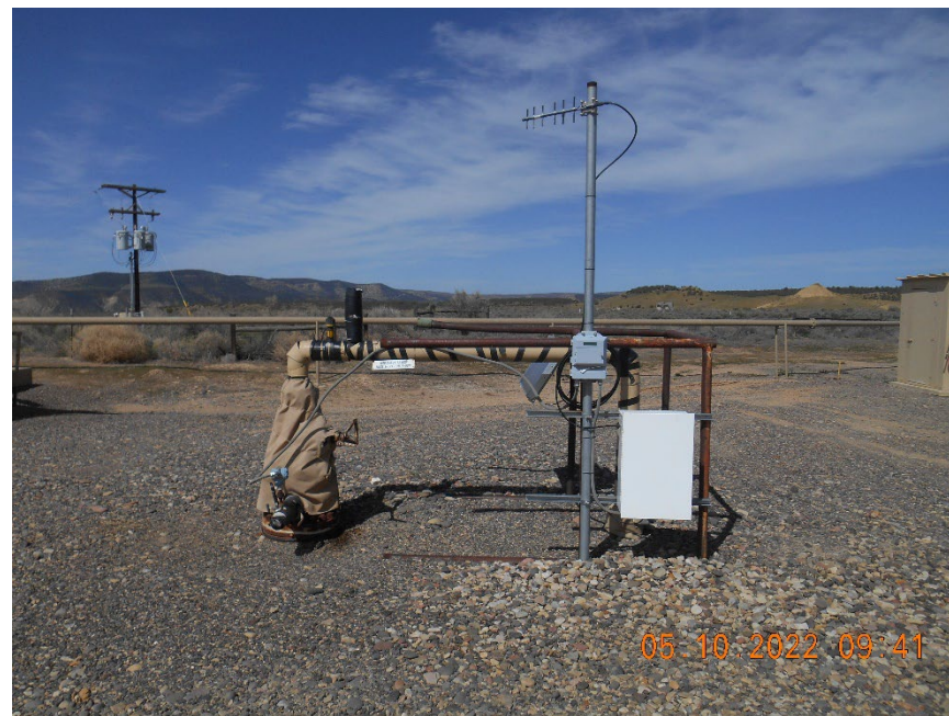
Injection wellhead
