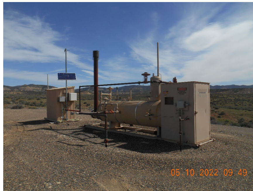
Separator and meter housing
