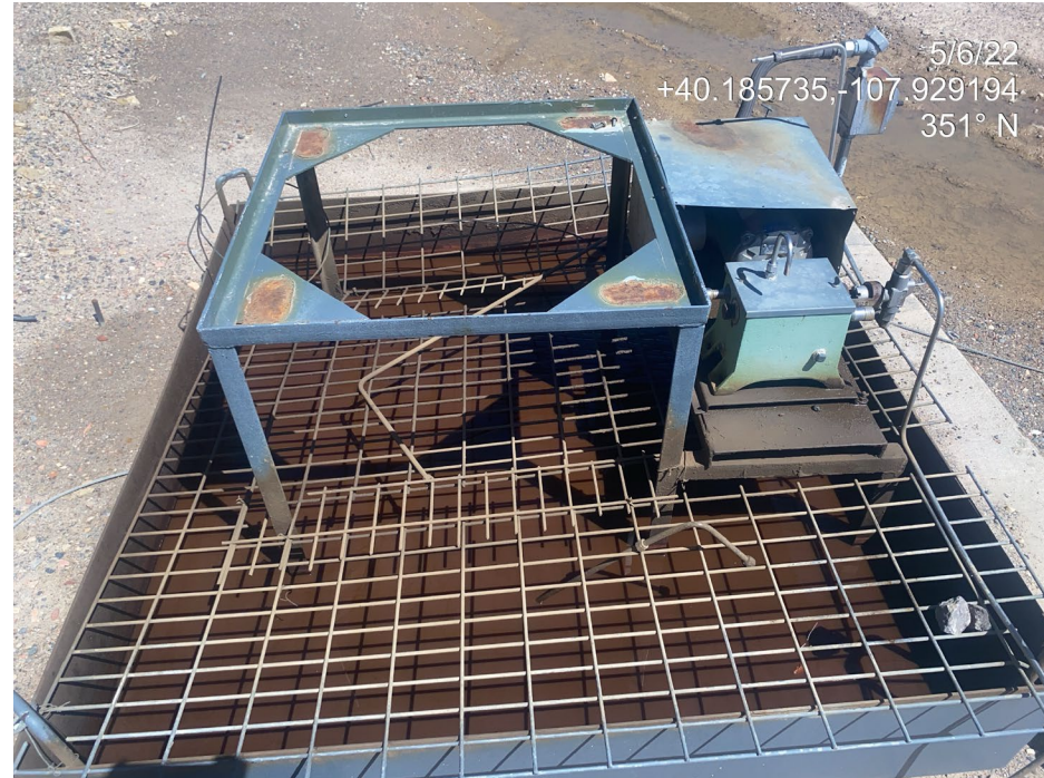
Photo 2. Photo shows a secondary containment BMP filled with fluid. Wildlife protection BMPs to enable wildlife egress are missing or insufficient.
