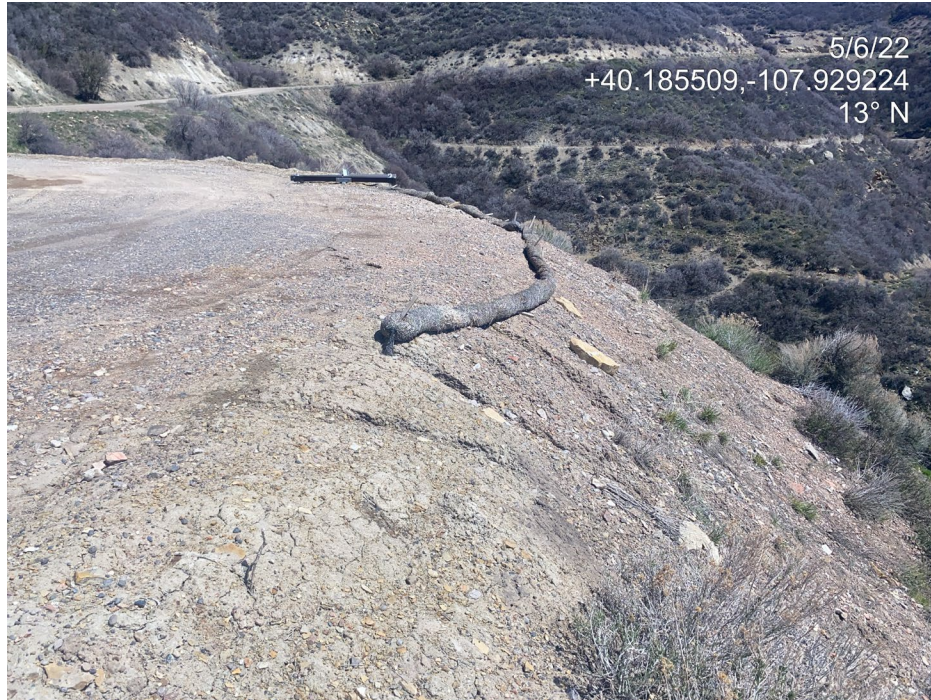
Photo 3. Photo taken from the east of the Location shows stormwater and sediment control BMPs are missing or insufficient. Erosion is evident on the eastern perimeter of the Location.
