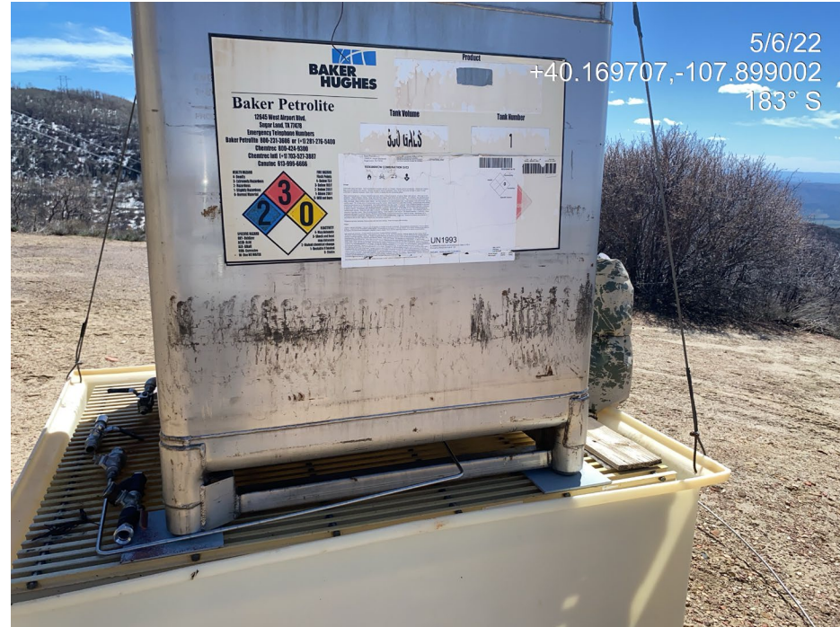
Photo 6. Photo shows a secondary containment BMP. Wildlife protection BMPs to enable wildlife egress were missing or insufficient.
