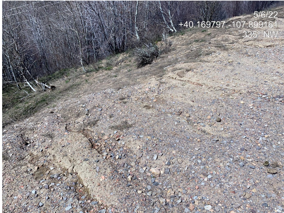
Photo 5. Photos taken from the western perimeter of the Location shows erosion occurring at the edge of the Location, resulting in transport of sediment offsite and offsite degradation.
