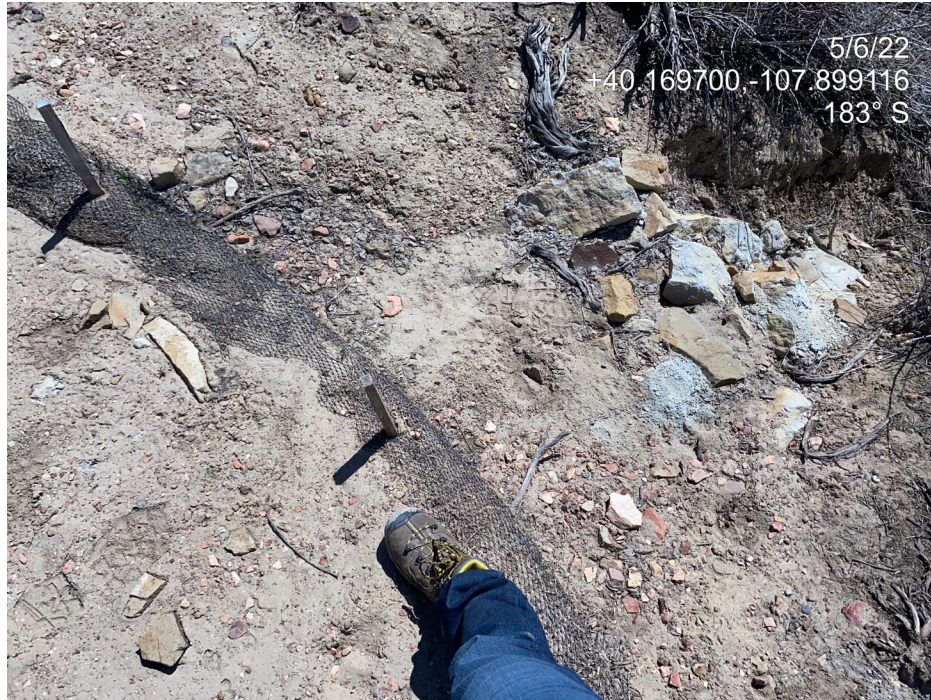
Photo 3. Photos taken from the western perimeter of the Location shows a straw wattle which is not in proper functioning condition to minimize erosion and transport of sediment offsite.
