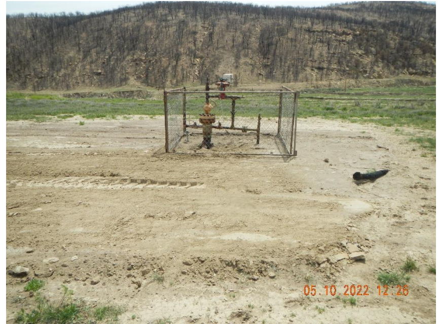
Hole in front of well has been back filled.
