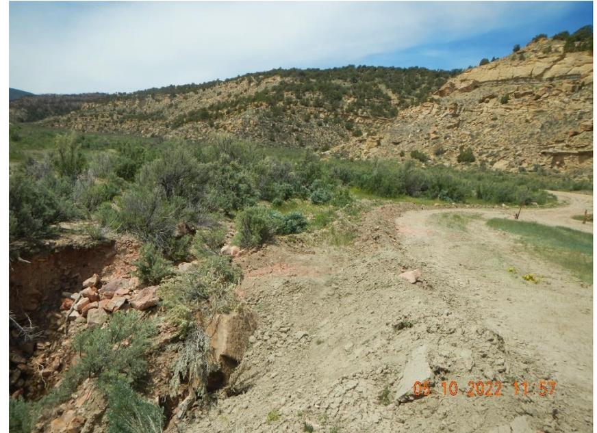
**Installed berm not compacted.**
