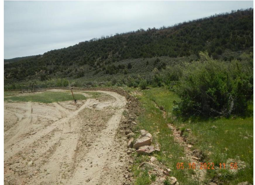
**Installed berm not compacted.**
