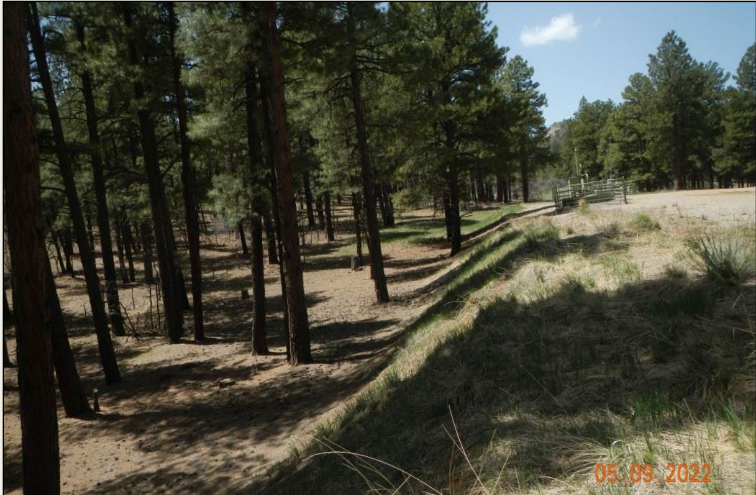
Photo 2. View of the southern fill slope from the southeastern corner facing westward. Revegetation is progressing largely with smooth brome, western wheatgrass, intermediate wheatgrass, and sand dropseed.
