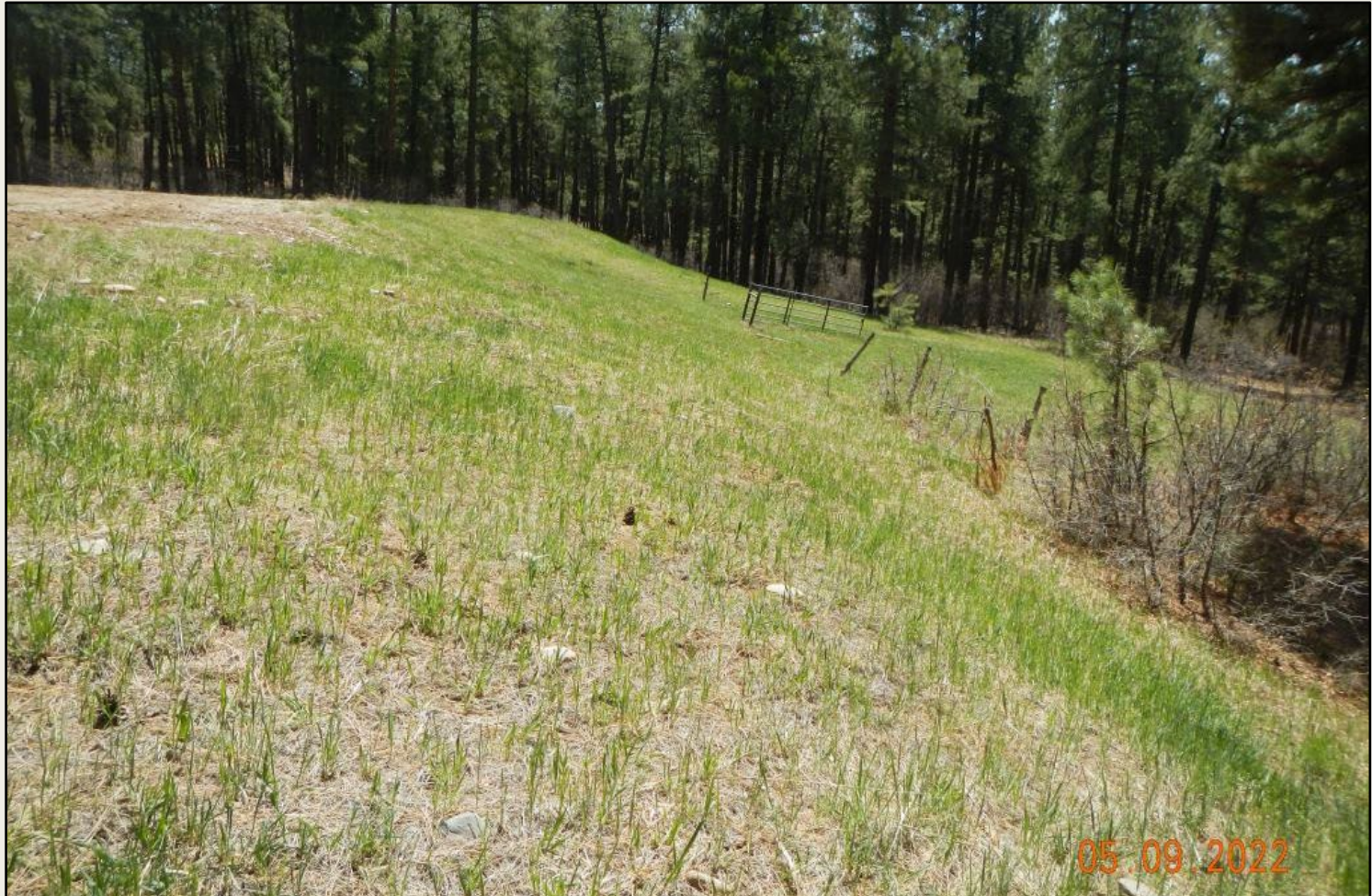
Photo 2. View of the western fill slope from the northwestern corner facing southward. Revegetation is progressing largely with smooth brome.
