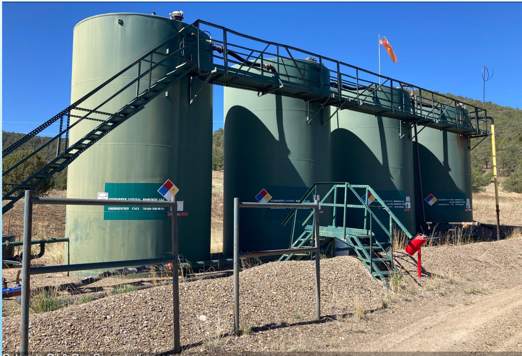
PHOTO 3: TANK BATTERY
