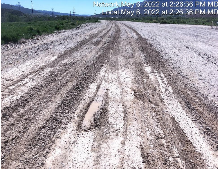
Photo #6637 Insufficient tracking BMP at entrance to location.
