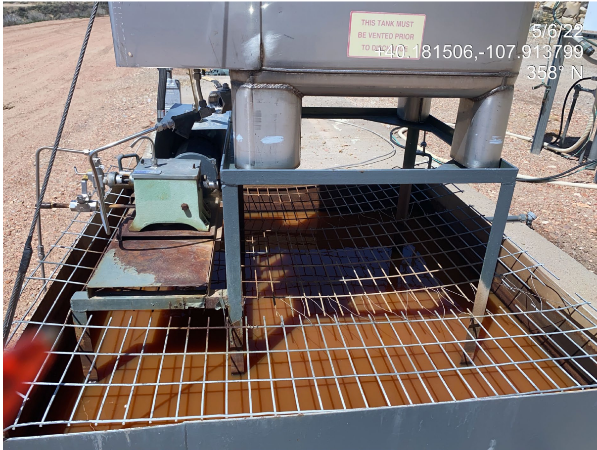
Photo 3. Photo shows a secondary containment BMP filled with fluid. Wildlife protection BMPs to enable wildlife egress are missing or insufficient.
