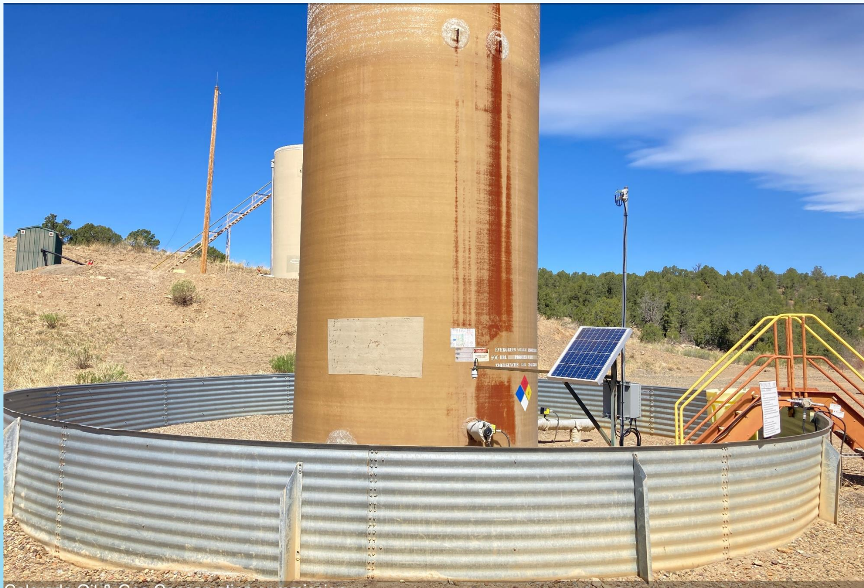
PHOTO 3: TANK BATTERY ON LOCATION
