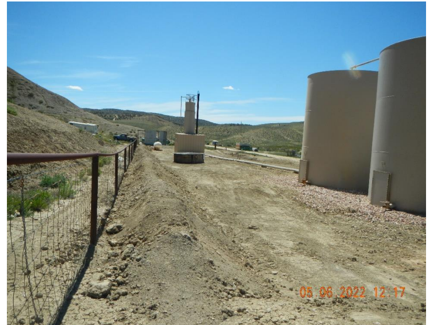
Tank berm repaired.
