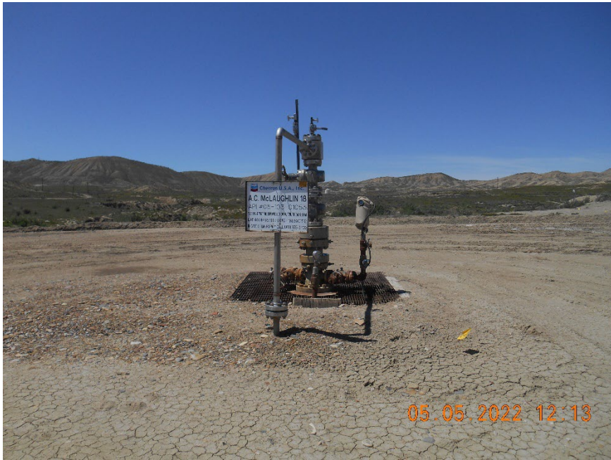
Injection wellhead
