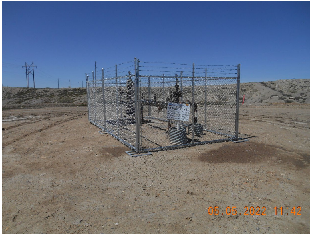
Injection wellhead
