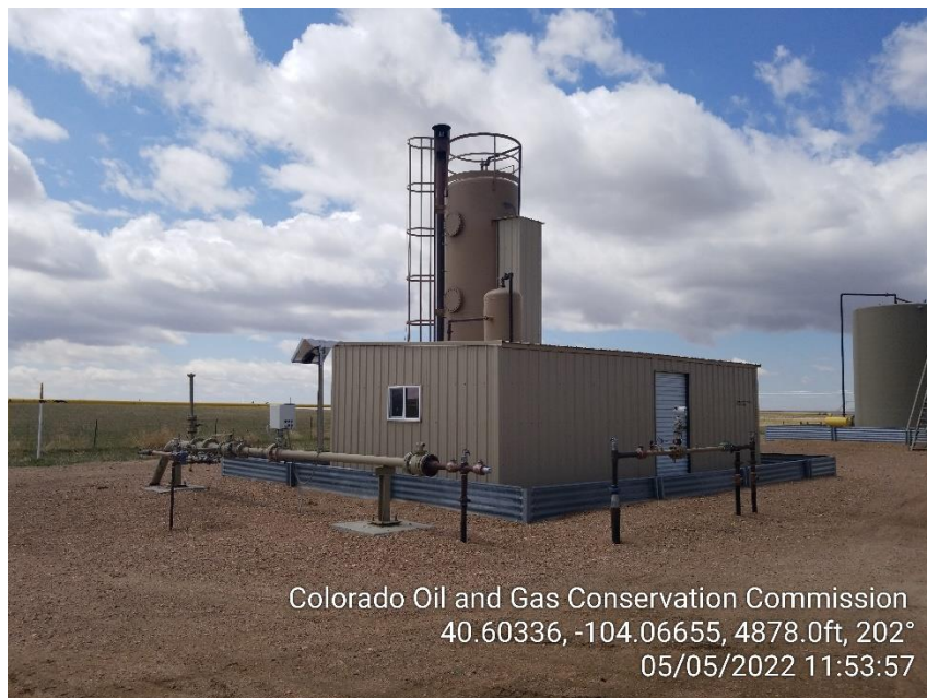
Photo 13 – Heater Treater and Gas Meters
