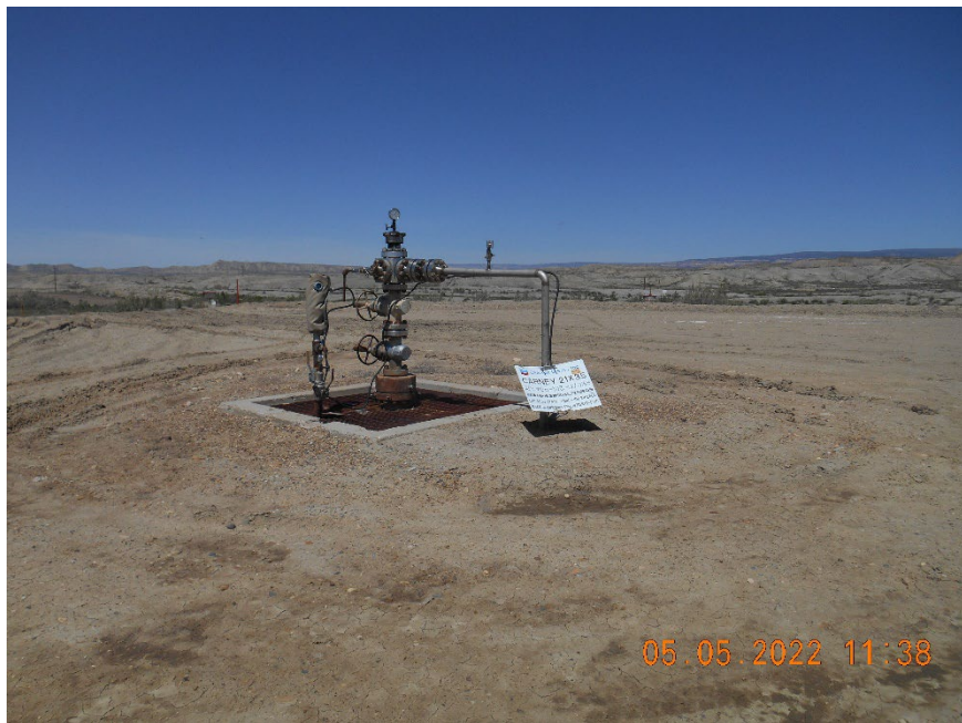
Injection wellhead
