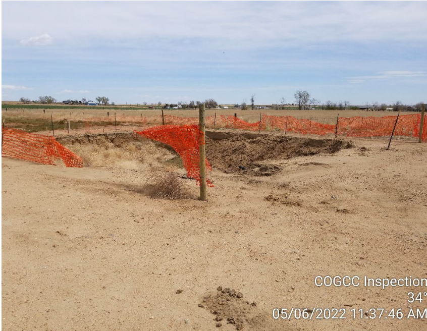
Photo 5 – Open excavation; fencing down.
