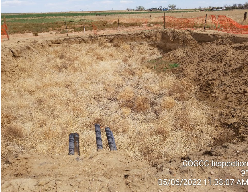
Photo 9 – Pipes sticking out of sidewall of open excavation.
