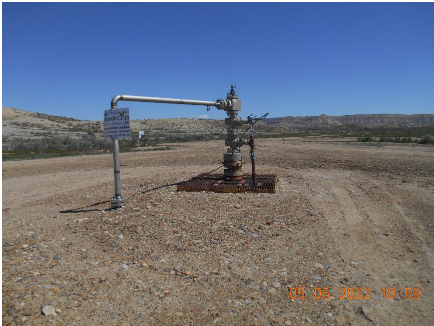
Injection wellhead
