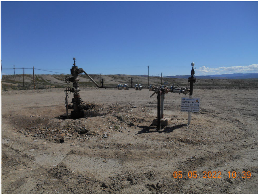
Injection wellhead
