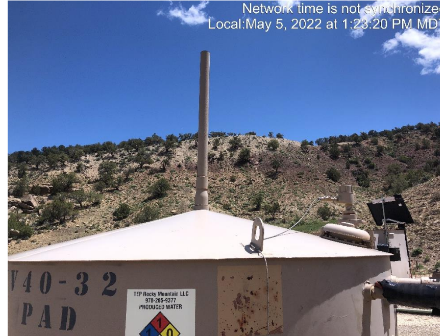
Photo #6620 Vent pipe on tank open ended.
