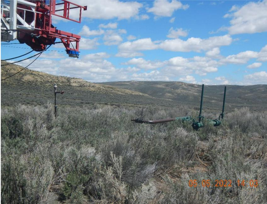
**Photo #8 flowline riser and gathering line riser to the east side of pad.**
