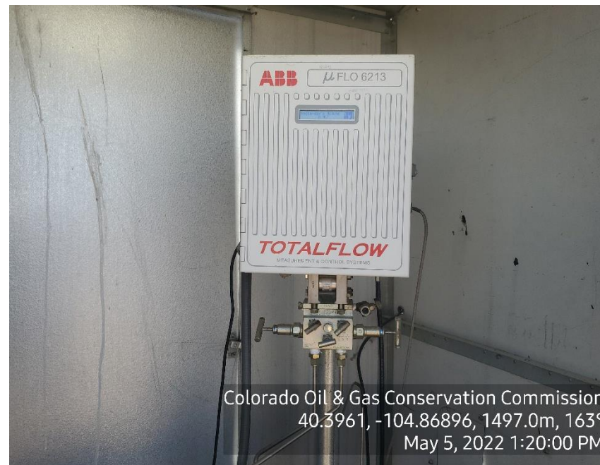
Photo 8: Calibration card not displayed
