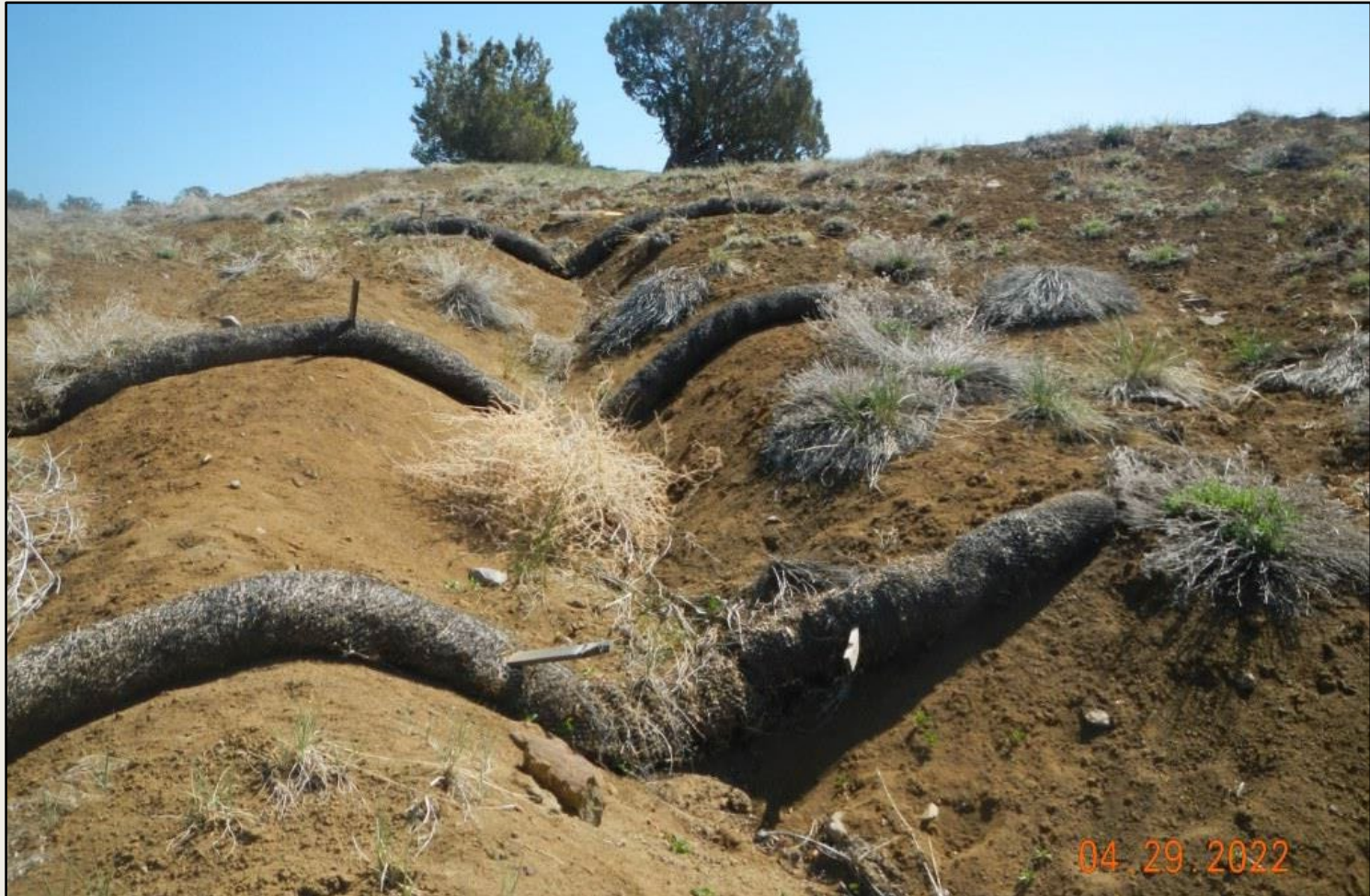
Photo 5. View of more erosional channeling forming within the southwestern project area. Wattles are not functioning and are not adequate BMPs for this area.
