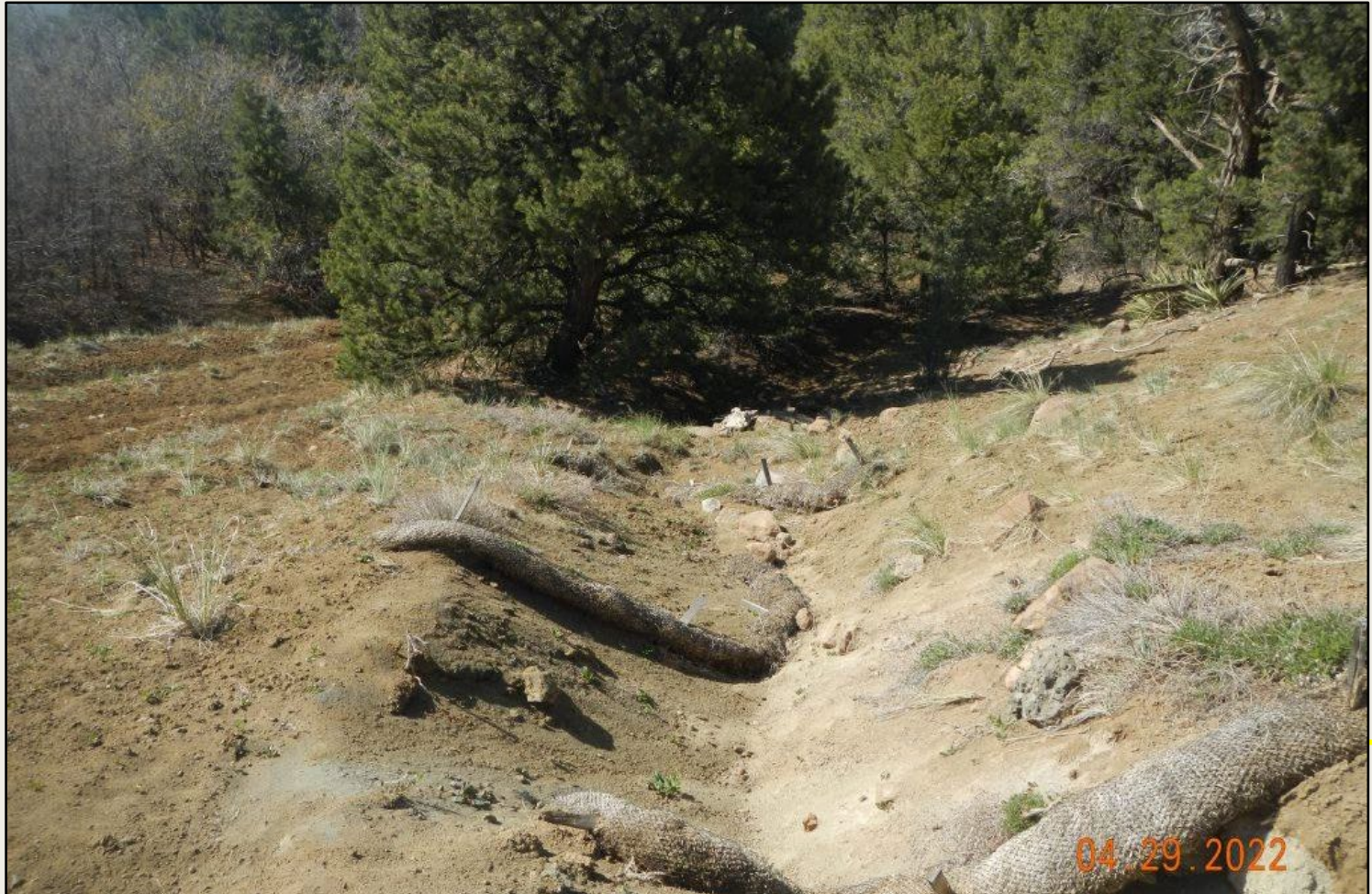
Photo 4. View of erosional channel forming within the southwestern project area. Wattles are not functioning and are not adequate BMPs for this area.
