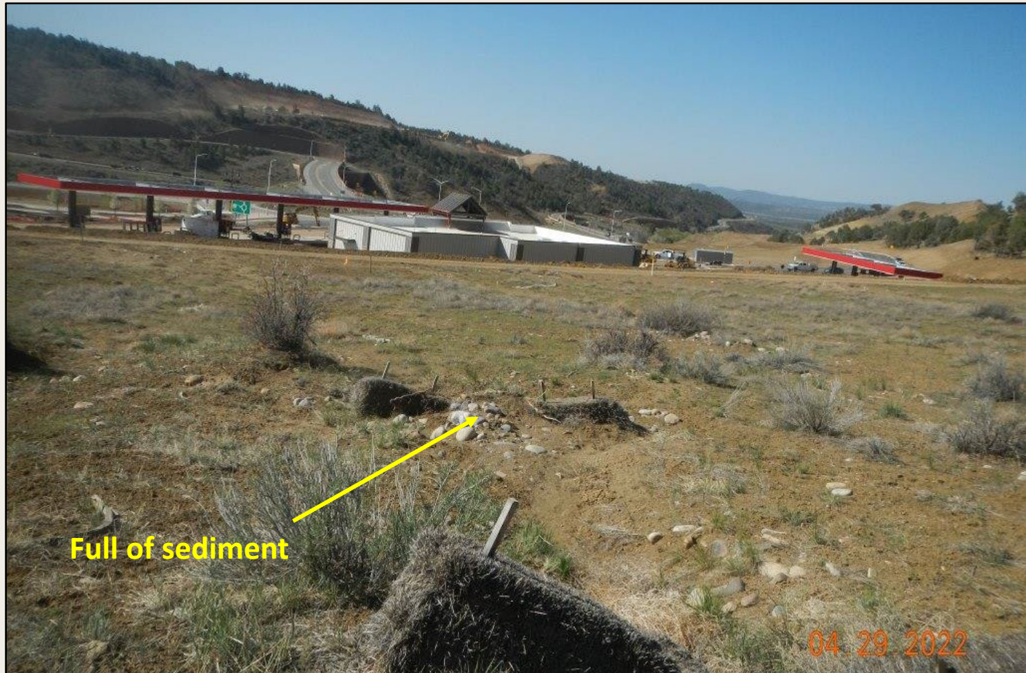
Photo 6. View of BMPs no longer functioning, where stormwater diversion is forming an erosional channel south of the project area.
