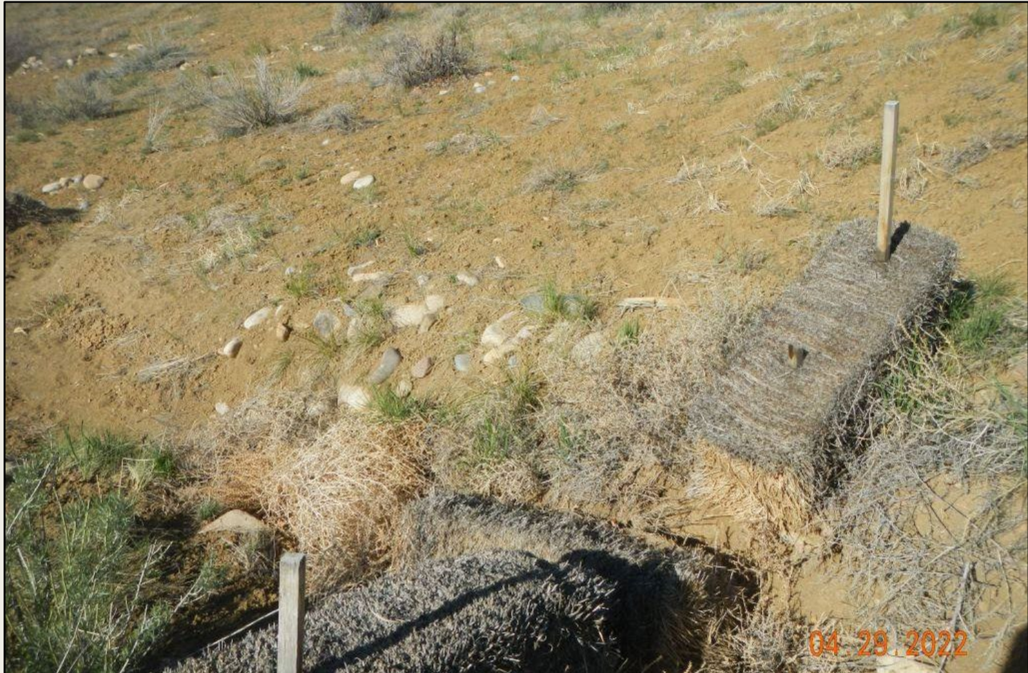
Photo 7. View of another BMP no longer functioning and not adequate in the southern project area.
