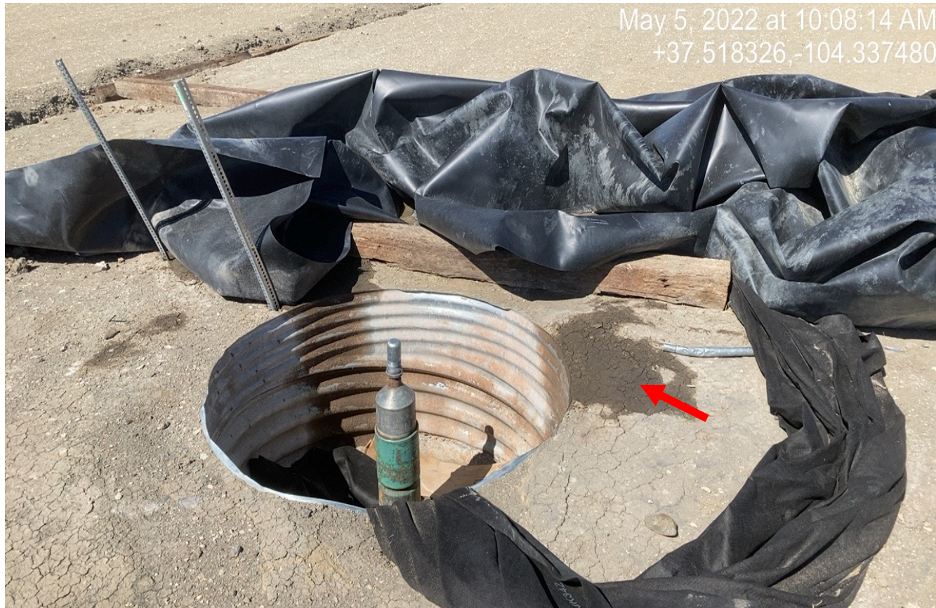
Photo 9. There are oil stained soils at the wellhead that needs to be cleaned up. The open top culvert and wellhead needs to be cover and protected to prevent wildlife entry.
