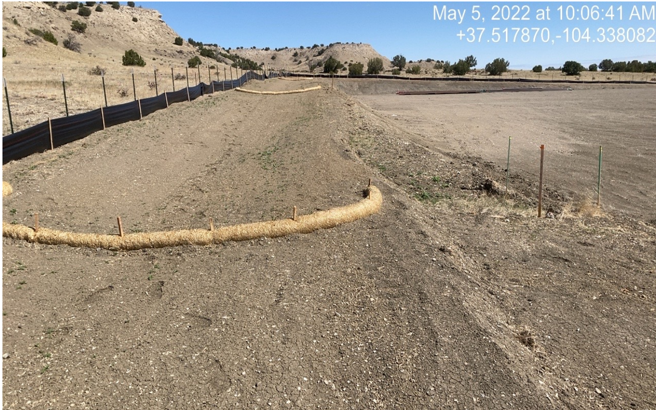
Photo 7. Southwest side of the location facing north. There are wattles installed along the perimeter swale.
