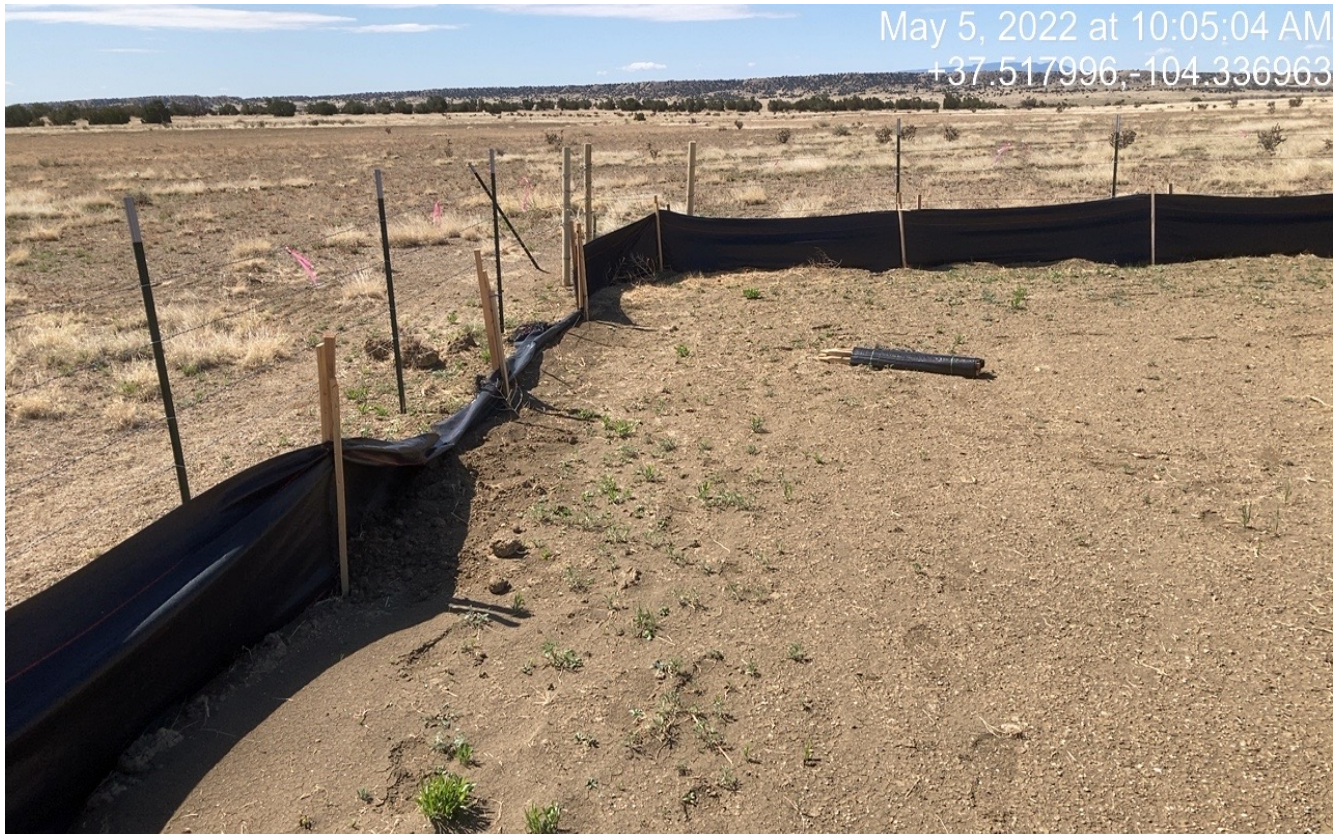
Photo 4. The silt fence at the southeast corner is in need of maintenance.
