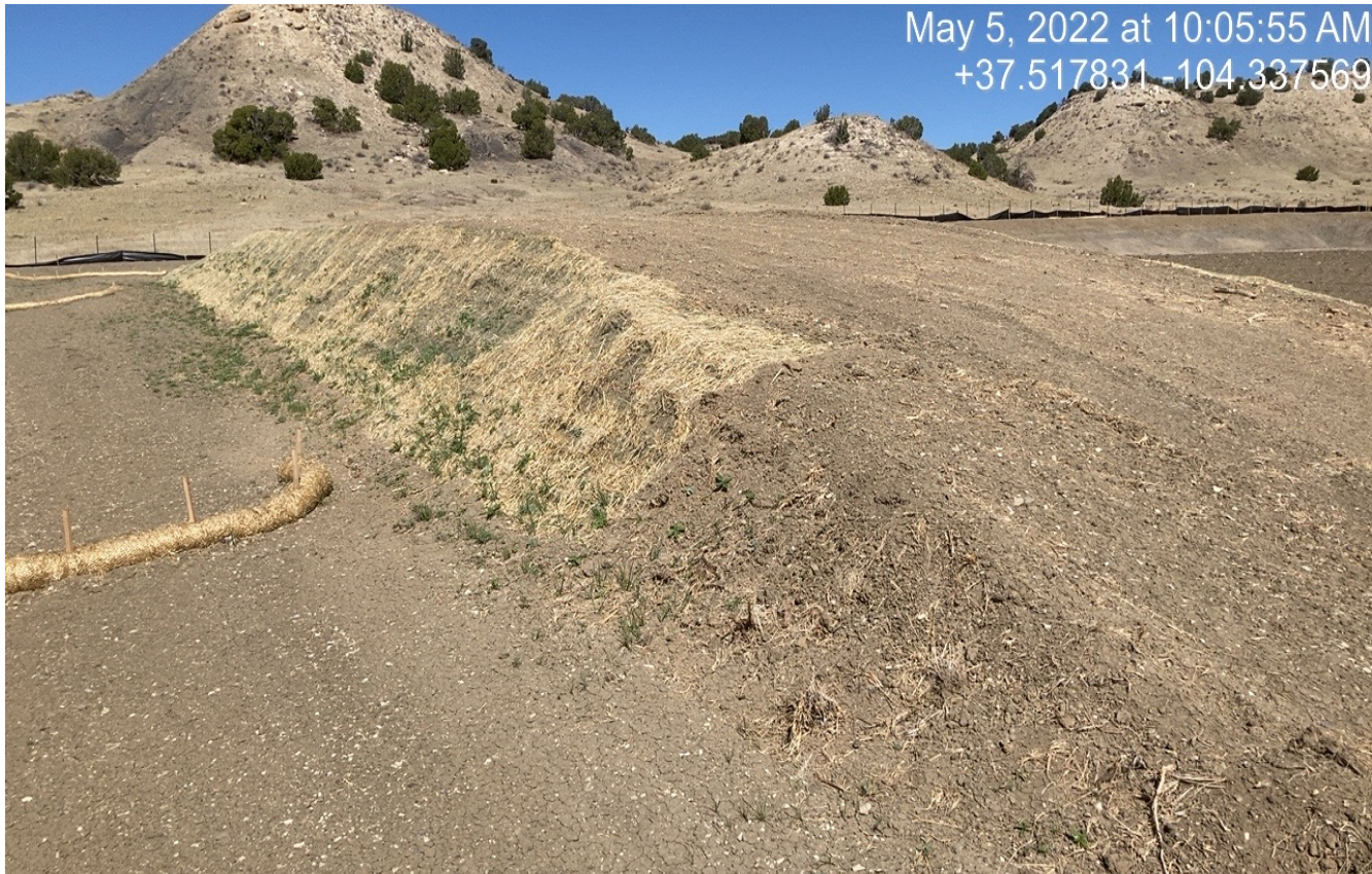
Photo 6. Facing toward the topsoil stock pile. There is blanket installed along the sides however the entire topsoil pile needs to be protected and maintained.
