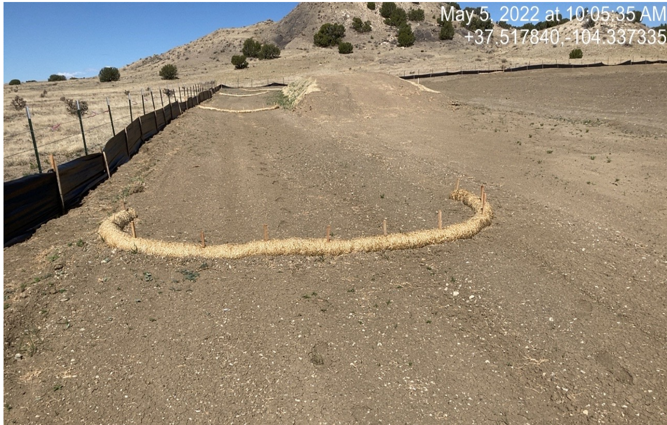
Photo 5. Facing west. There are wattles installed along the perimeter swale.
