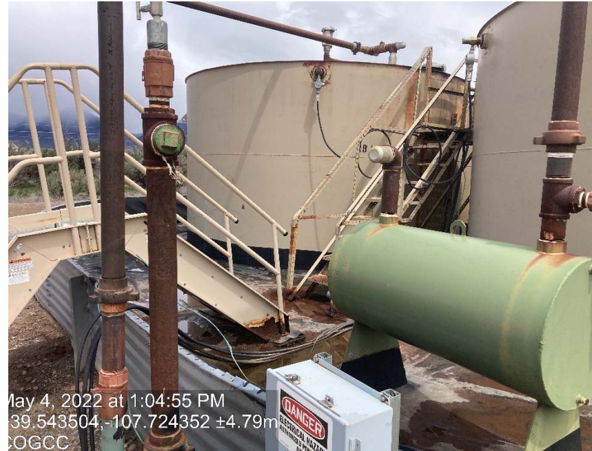
Line to ECD is disconnected at tanks
