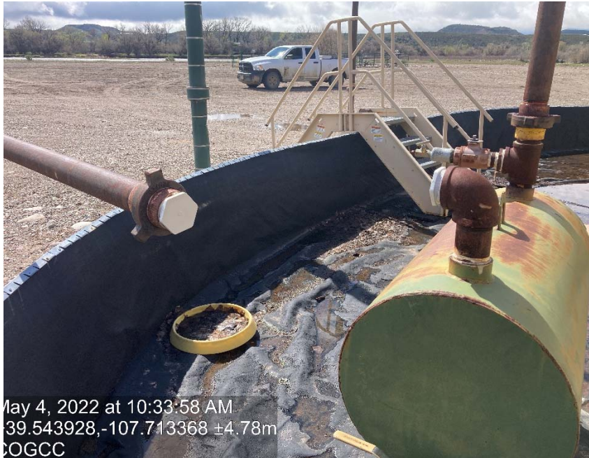
Line to combustor (ECD) disconnected at tanks
