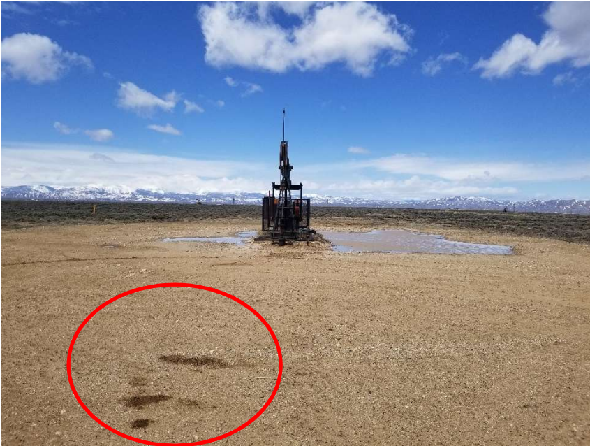
Photo 1. Overview of location taken facing northwest. Stained soil on location.
