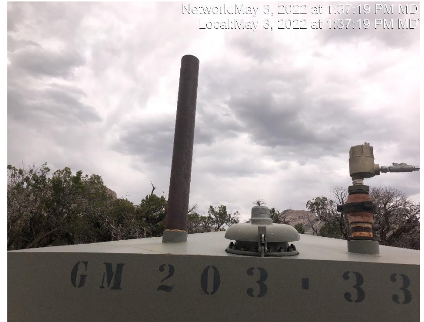
Photo #6603 Vent pipe on tank open ended.
