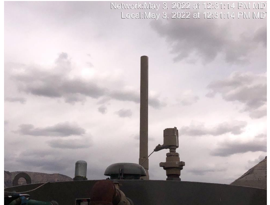
Photo #6598 Vent pipe on tank open ended.
