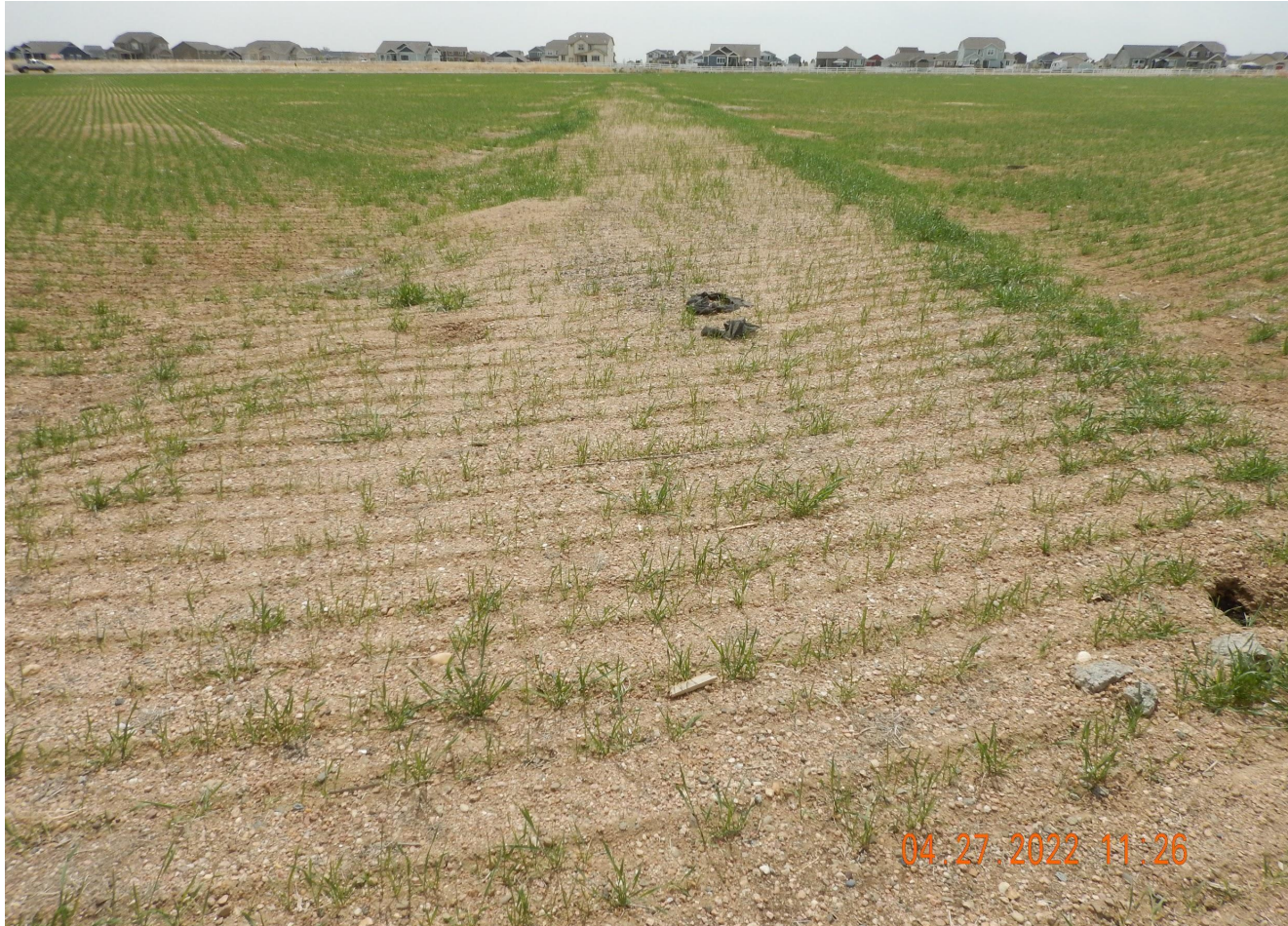
Photo 1. Photo taken from the northern well location access road, facing South. Photo illustrates Operator has failed to comply with Rule 1004 standards and has not removed gravel, recontour and perform subsequent final reclamation (i.e., compaction alleviation, etc..).
