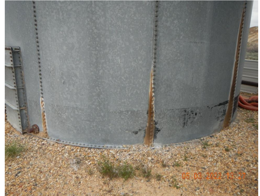
Stains around tank's bolted seams.
