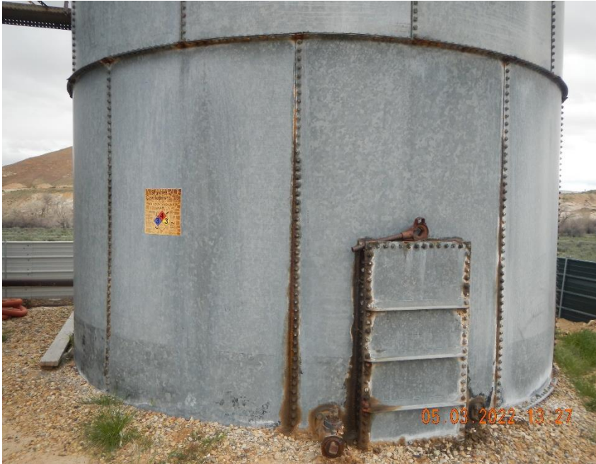
Stains around tank's bolted seams.
