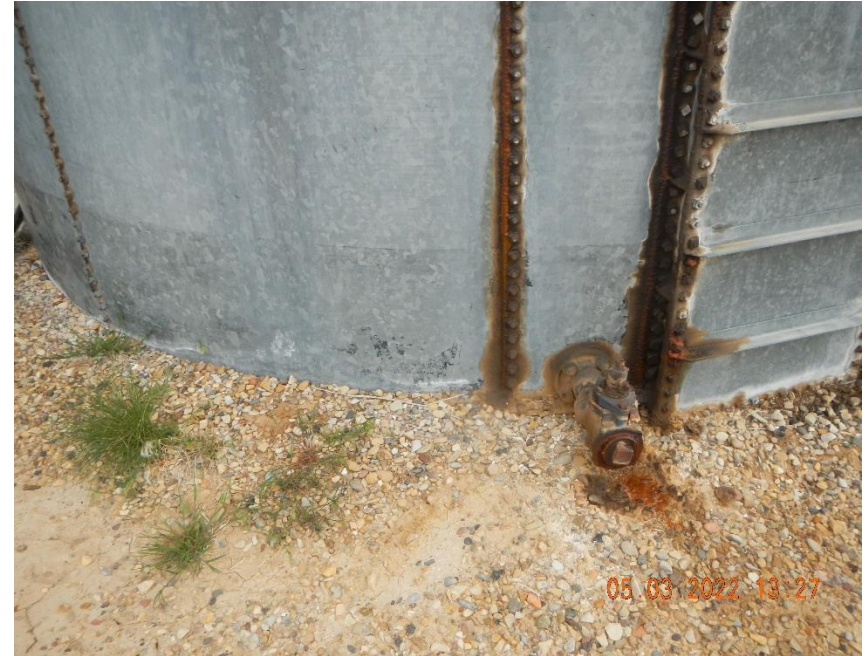
Crude oil stains at product valve on tank.
