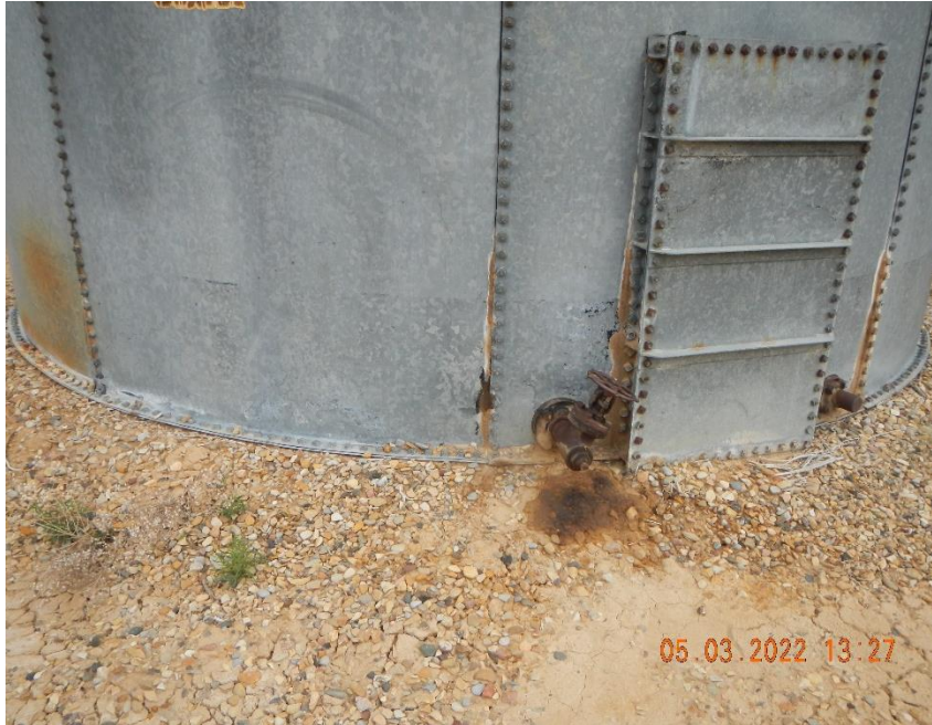
Crude oil stains at product valve on tank.
