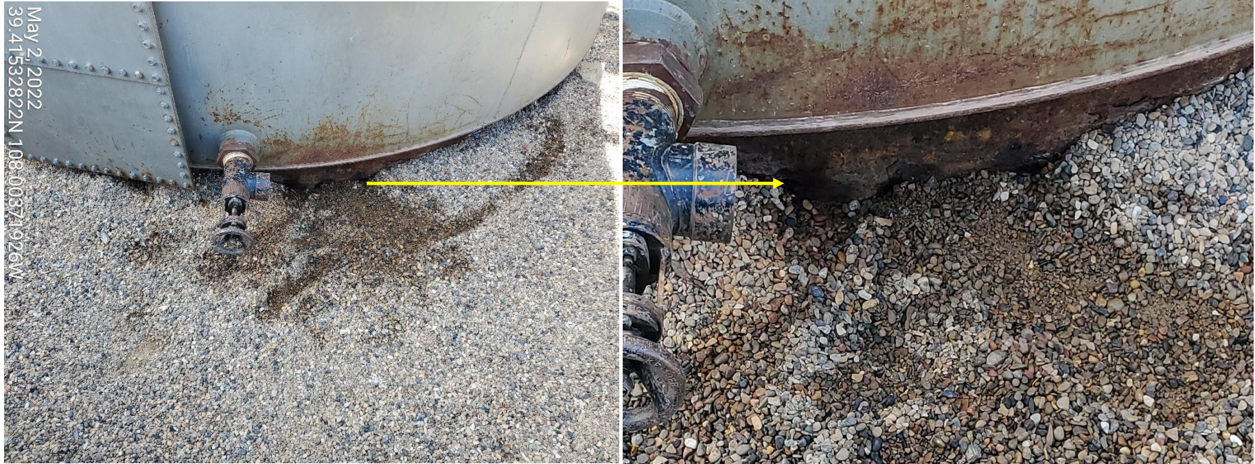
Photo 9: Photos taken from the northeastern-most condensate tank on the Location. Photo shows rusting and possible integrity issues at the base of the tank, as well as stained soils within the same area.
