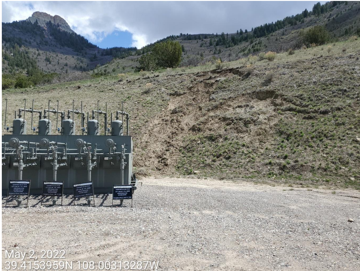
Photo 3: Photo taken from the southeast end of the Location, facing west. Photos 3-8 show areas along the slopes on the south end of the Location, where erosion degradation resulting in mass soil migration from the slopes is evident. Areas require additional reclamation and stabilization.
