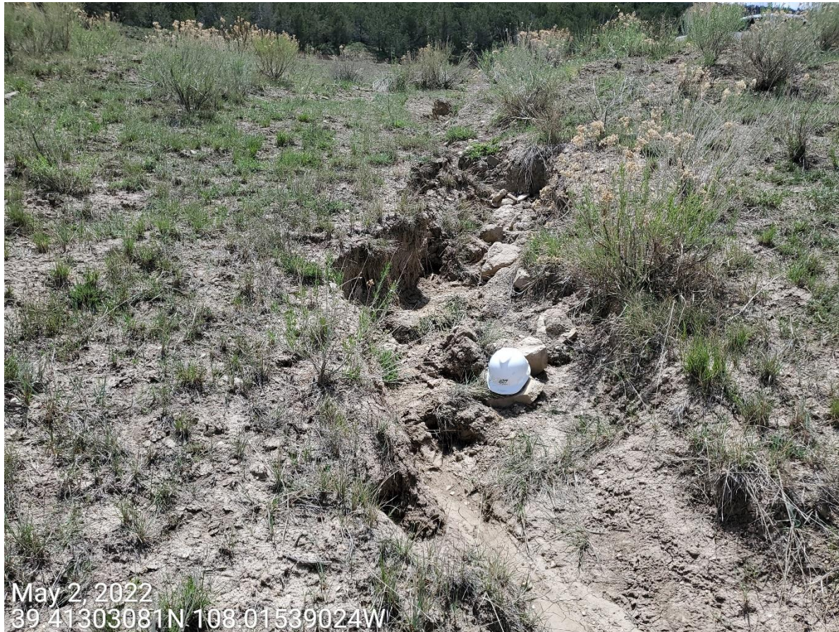
Photo 4: Photo taken from the north end of the Location. Photo shows erosion degradation at the sediment trap control measure. Hard hat used for reference.
