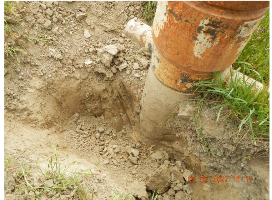
Casing has been dug around.
