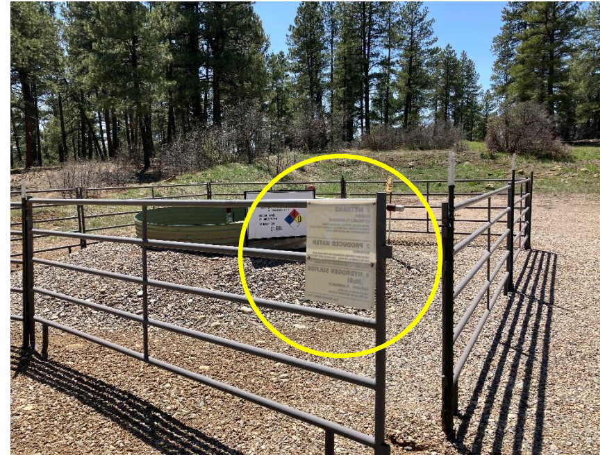
IMG-0013, Produced water tank placard facing inward
