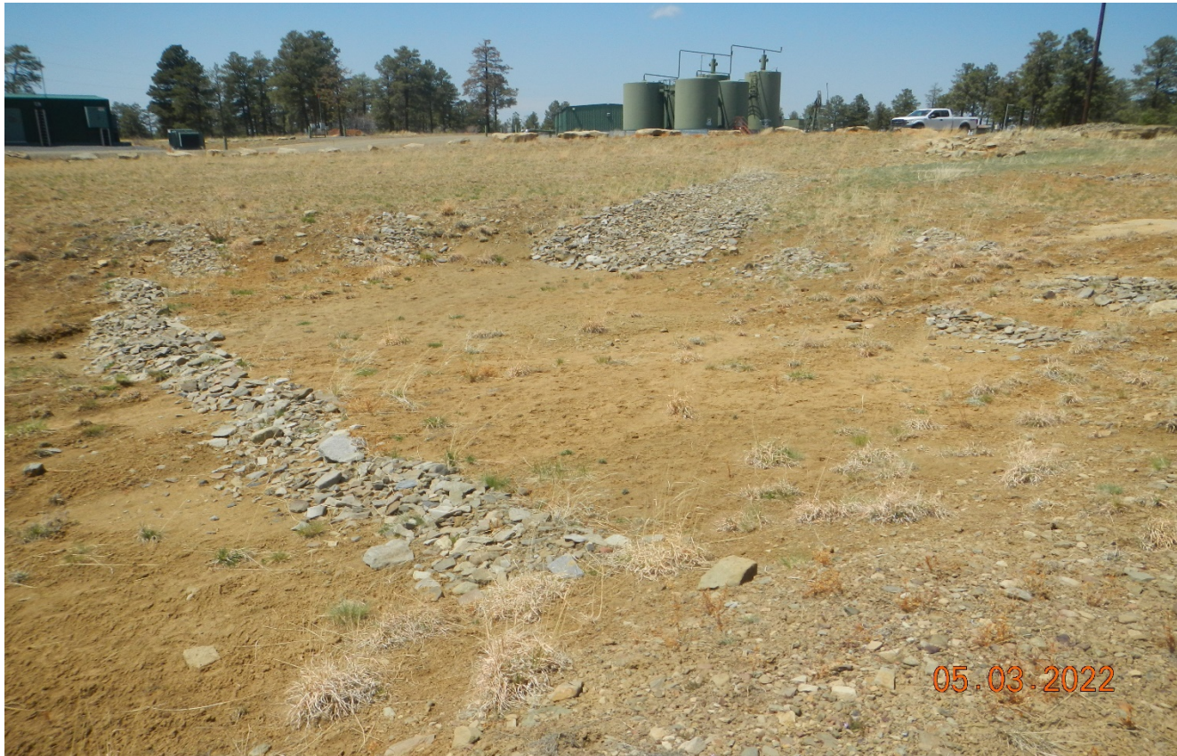
Photo 3. Facing west at the location. There are rock check dams installed where erosion was occurring. This area could use additional hand seeding to establish vegetation.
