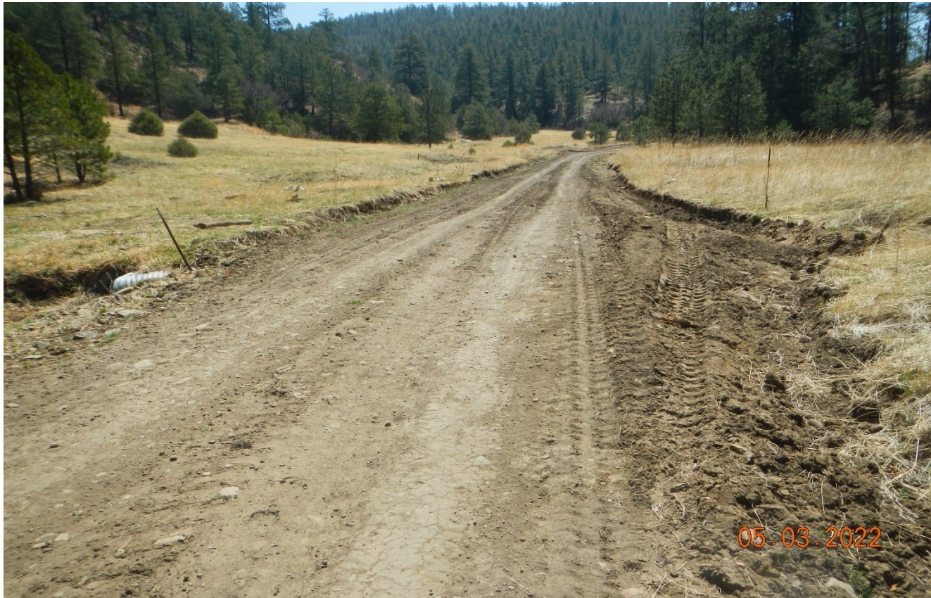
Photo 3. The culvert along the road is filled in with sediment causing stormwater to flow down the side of the road. Lat/Long:37.00499,-104.83742. Previous corrective action was not completed.
