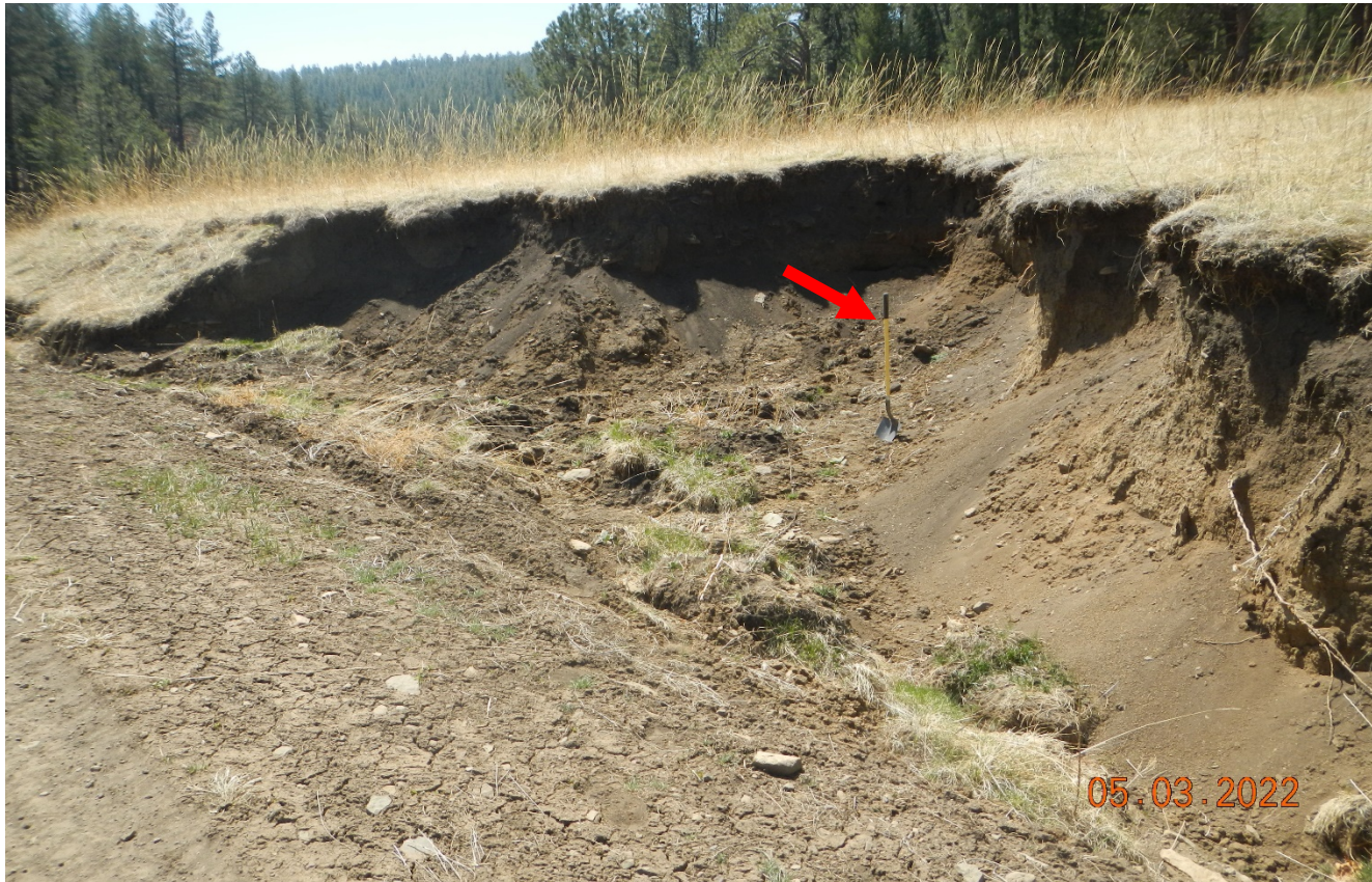
Photo 6. The side of the road is eroded and not stabilized at Lat/Long:36.99952,-104.83425. Erosion head cutting is continuing to occur further back. This area needs to be repaired and stabilized. Previous corrective action not completed. Red arrow points to 4.5 ft. shovel.
