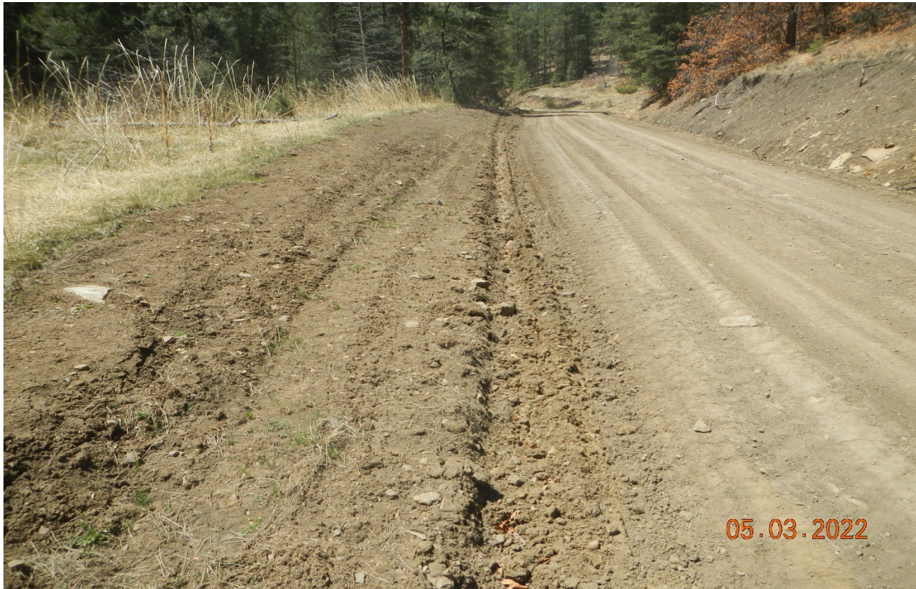
Photo 7. There was grading performed along the road. The disturbance along the side of the road needs to be seeded and reclaimed. Previous corrective action not completed.
