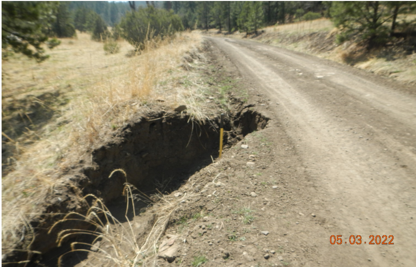
Photo 4. There is an erosion gully along the road that needs to be repaired and stabilized.
