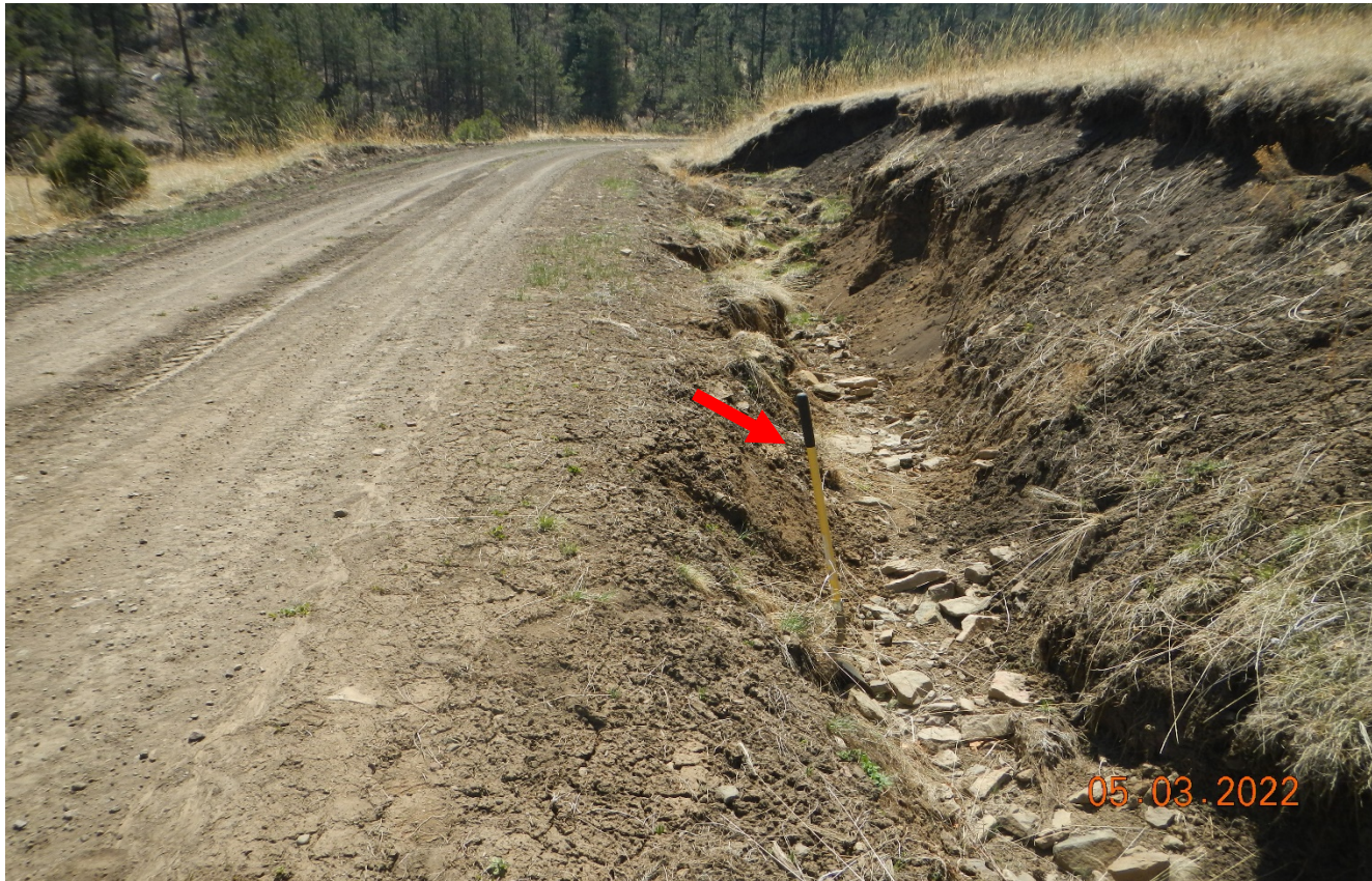
Photo 5. The side of the road is eroded and is not stabilized at Lat/Long:36.99952,-104.83425. This area or erosion needs to be repaired and stabilized. Previous corrective action not completed. Red arrow points to 4.5 ft. shovel.
