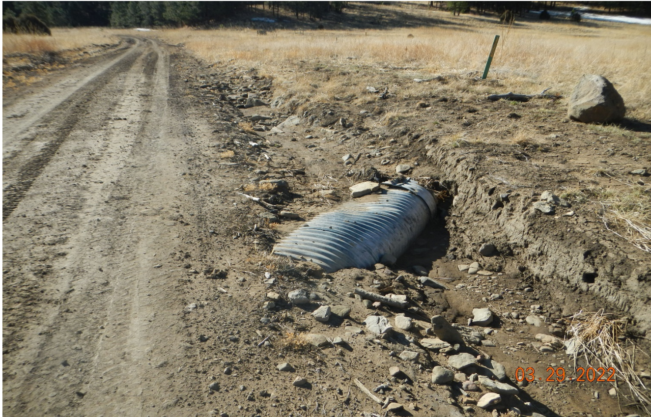
Photo 2. The culvert along the road is filled in with sediment causing stormwater to flow down the side of the road. Lat/Long:37.00581,-104.83861. Previous corrective action was not completed.
