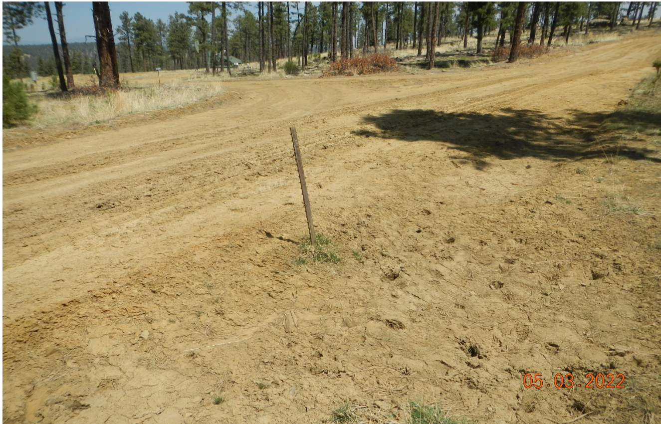
Photo 8. The culvert along the road is filled in with sediment at Lat/Long:36.99405,-104.84710. Previous corrective action not completed.
