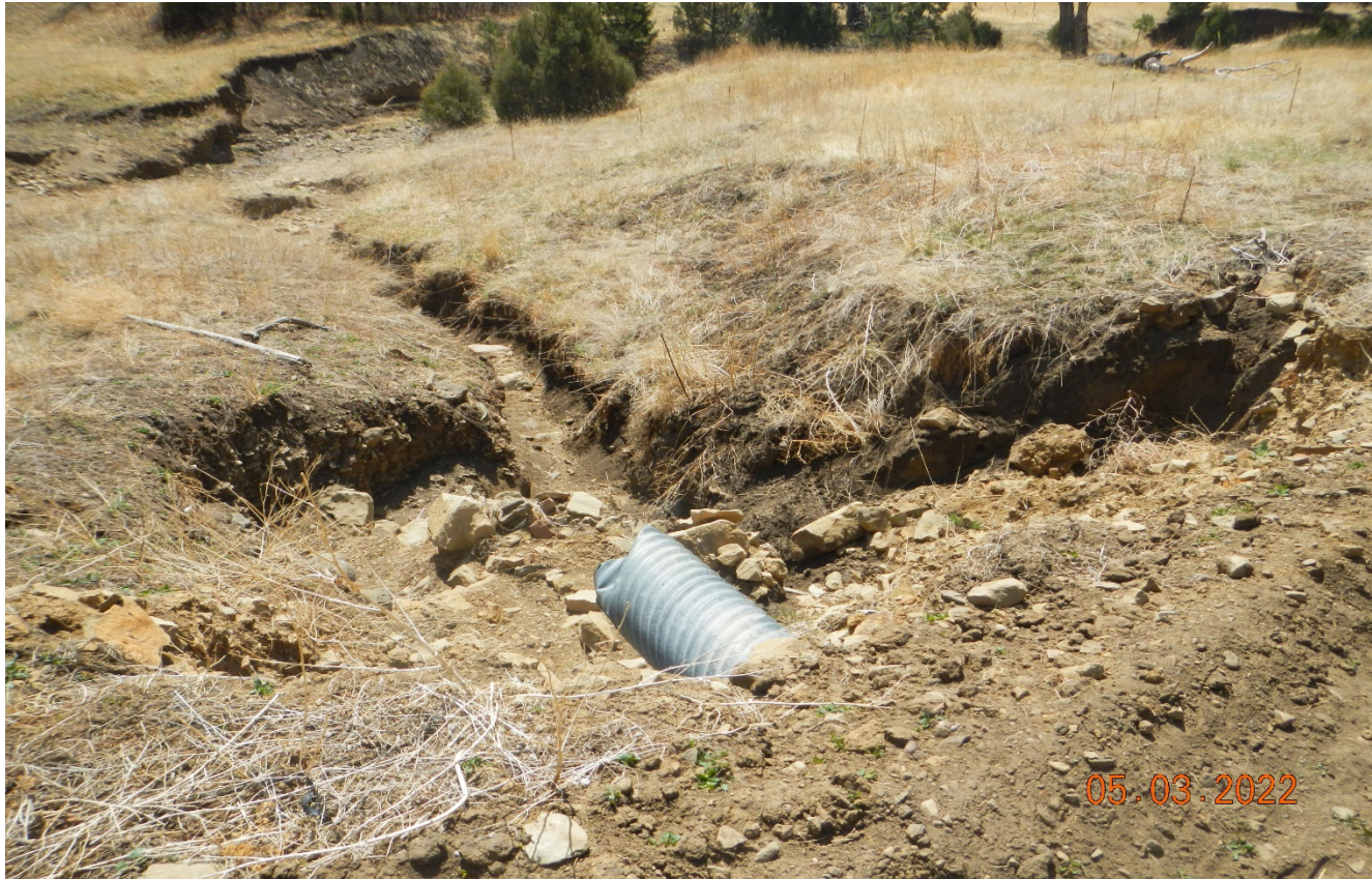
Photo 2. The culvert outlet is eroded and does not have outlet protection. Previous corrective action not completed.
