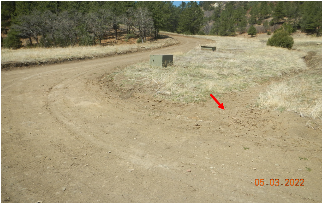
Photo 1. Facing west toward the access road ascending the hillside. The road has been graded. The culvert inlet shown at red arrow is filled in with sediment. The culvert outlet is shown in photo 2.
