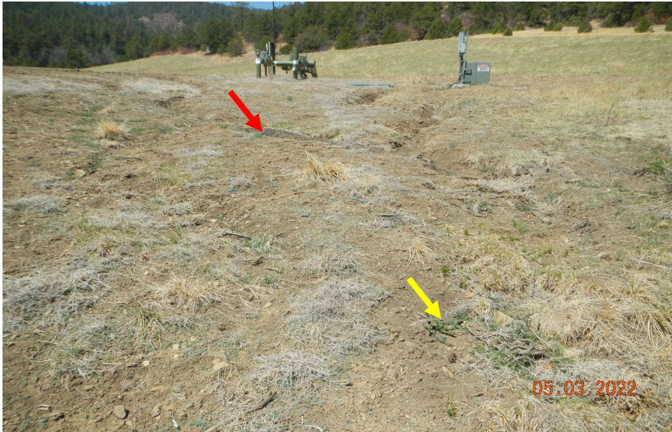
Photo 4. Facing toward the northeast side of the location. This area is not stabilized and there is an erosion. The wattles are degraded shown at red arrow. Previous corrective action not completed. There are noxious weeds beginning to grow (Yellow arrow – Musk thistle)
