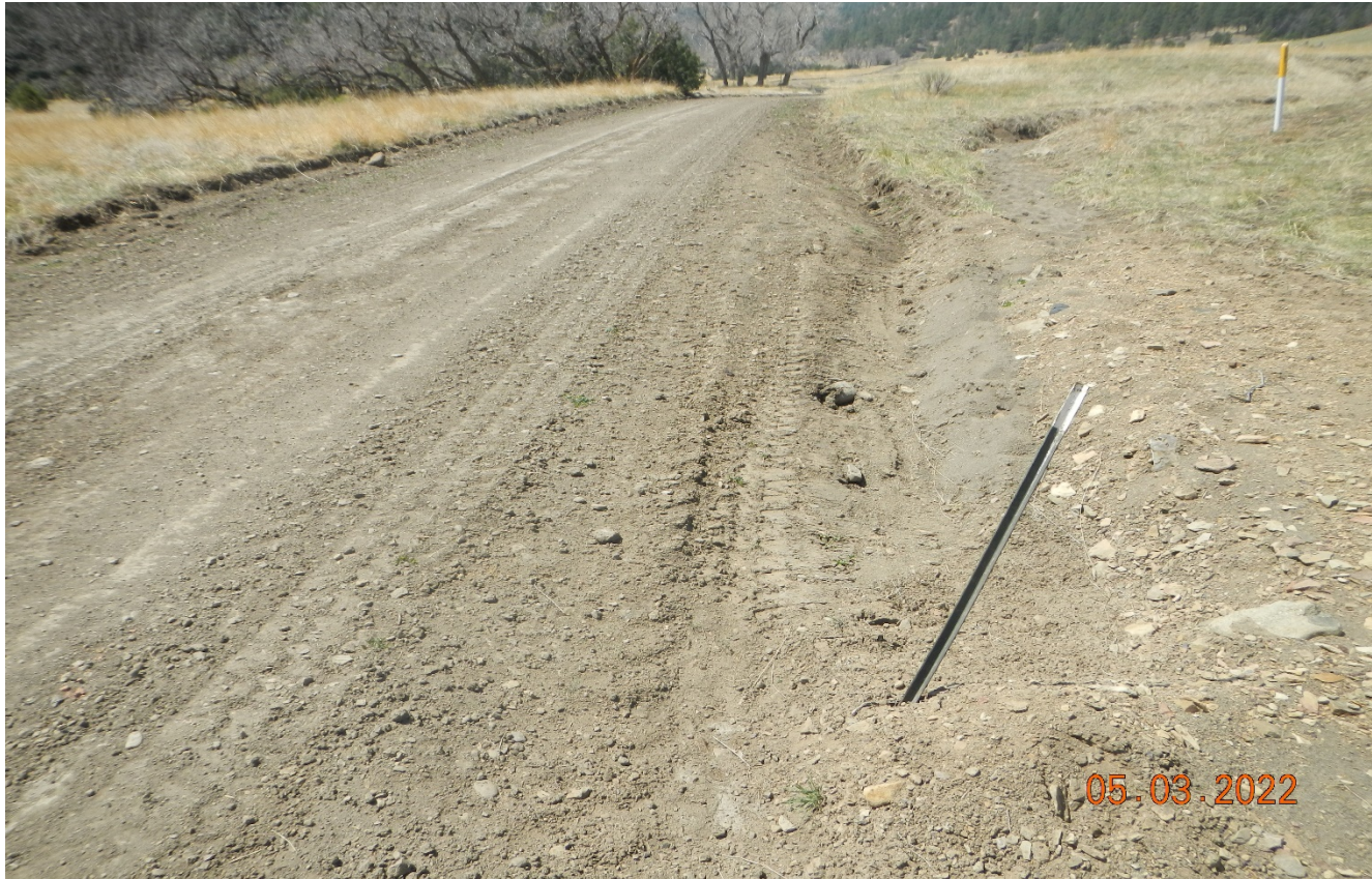
Photo 2. Facing southwest along the main road near the well site. Stormwater has washed across the road causing erosion. The culvert is filled in with sediment and has not been repaired. Previous corrective action not completed.
