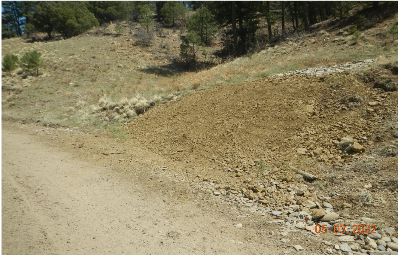
Photo 5. Facing southeast along the road. This area of erosion has been repaired but needs to be seeded and stabilized.
