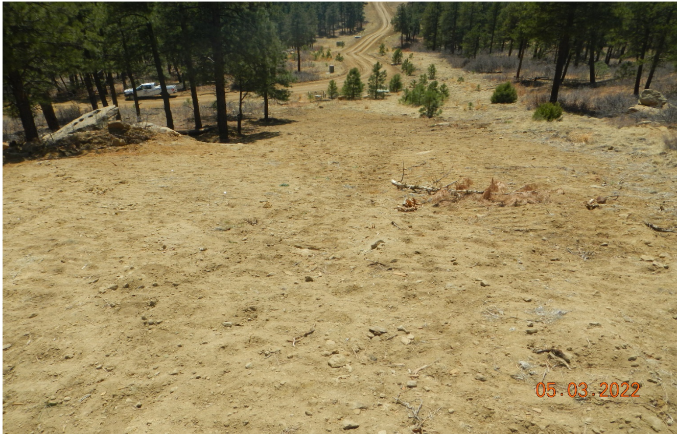
Photo 2. Facing southwest along the pipeline disturbance. The disturbed soils are susceptible to erosion and need to be seeded and stabilized.
