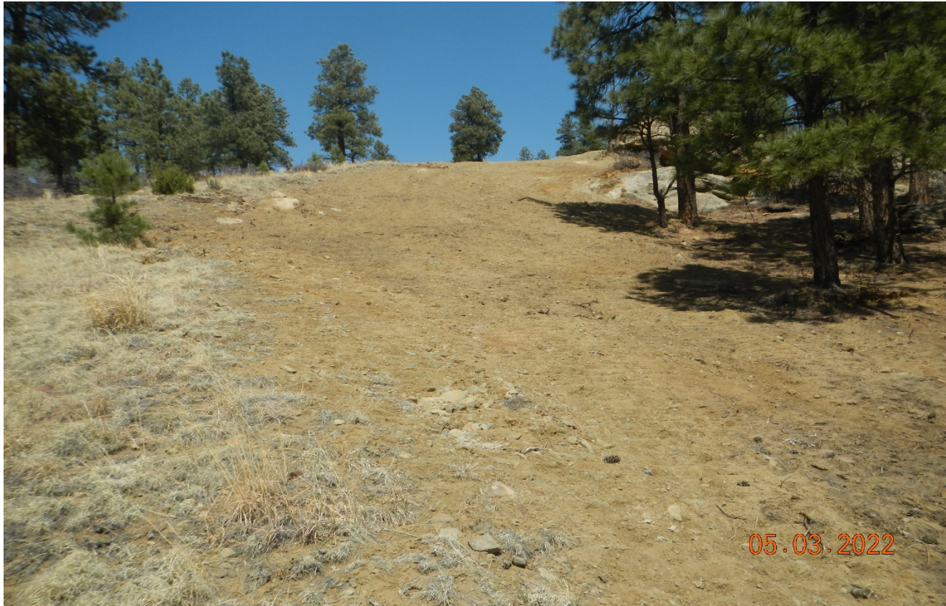
Photo 1. Facing northeast. There has been recent disturbance along the gathering pipeline at Lat/Long:37.05440,-104.76614.This area needs to be reclaimed and stabilized.
