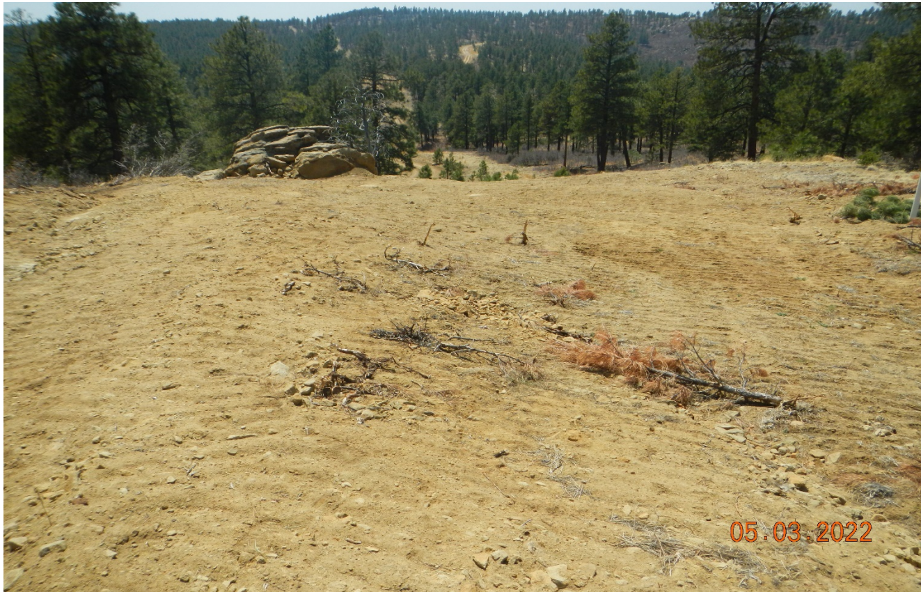
Photo 3. Facing southwest along the pipeline disturbance. The disturbed soils are susceptible to erosion and need to be seeded and stabilized.
