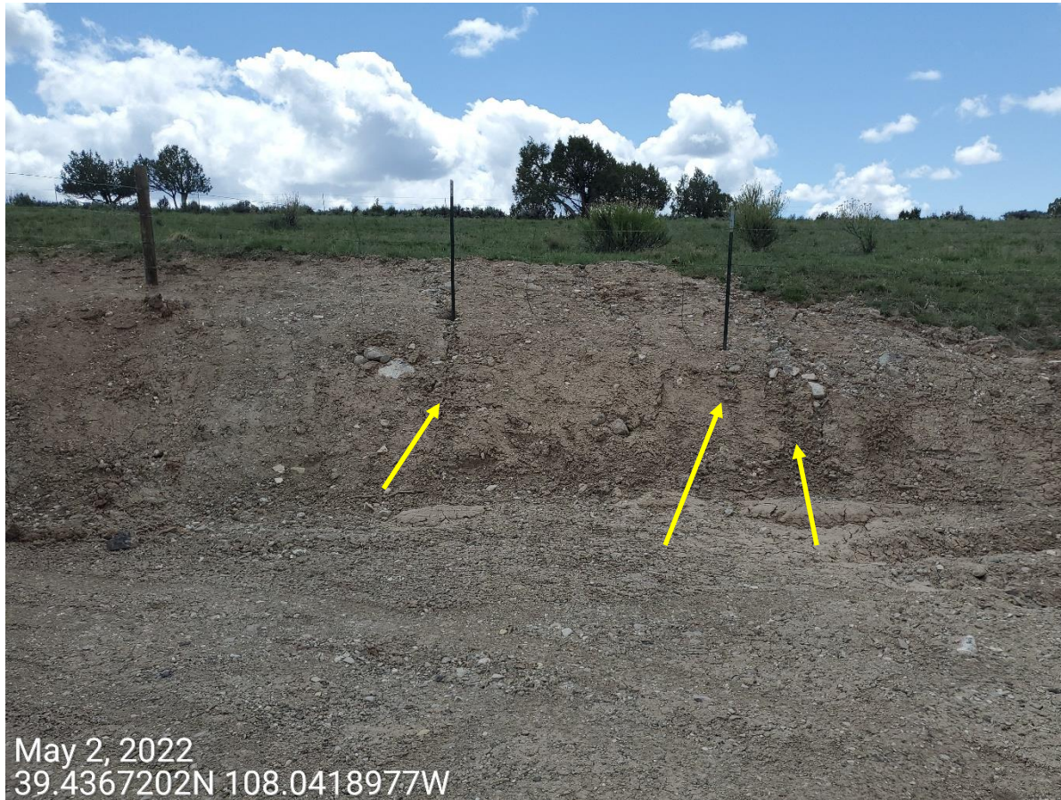
Photo 5: Photo taken from the cut slopes on the north end of the Location. Control measures to minimize erosion missing or insufficient at the cut slopes; erosion degradation observed.
