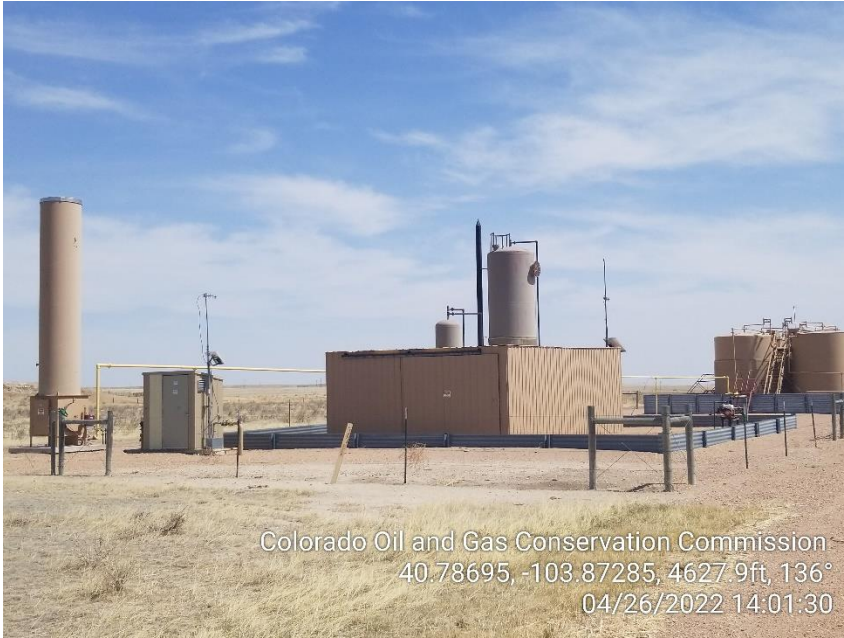
Photo 3 – ECD, Gas Meter and Heater Treater
