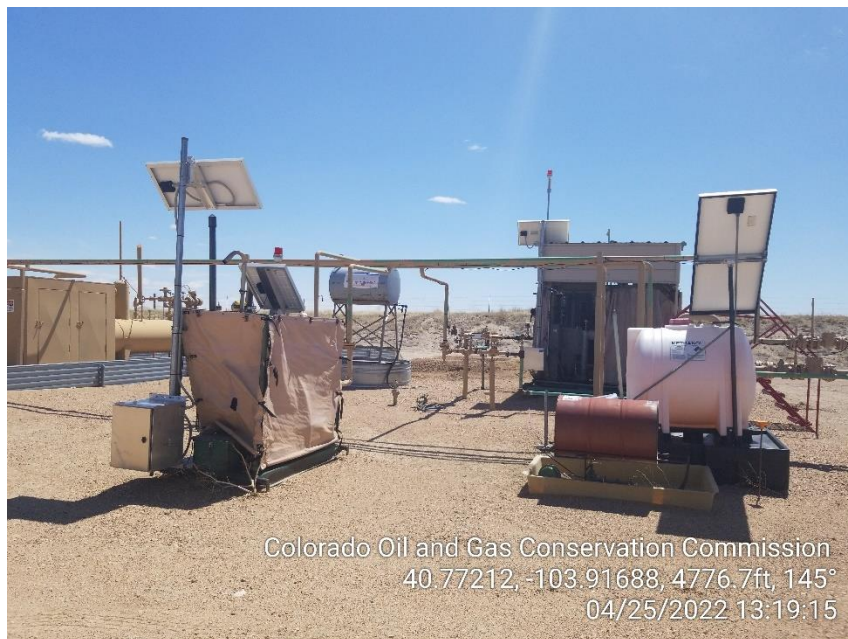
Photo 5 – VRU and Compressor
