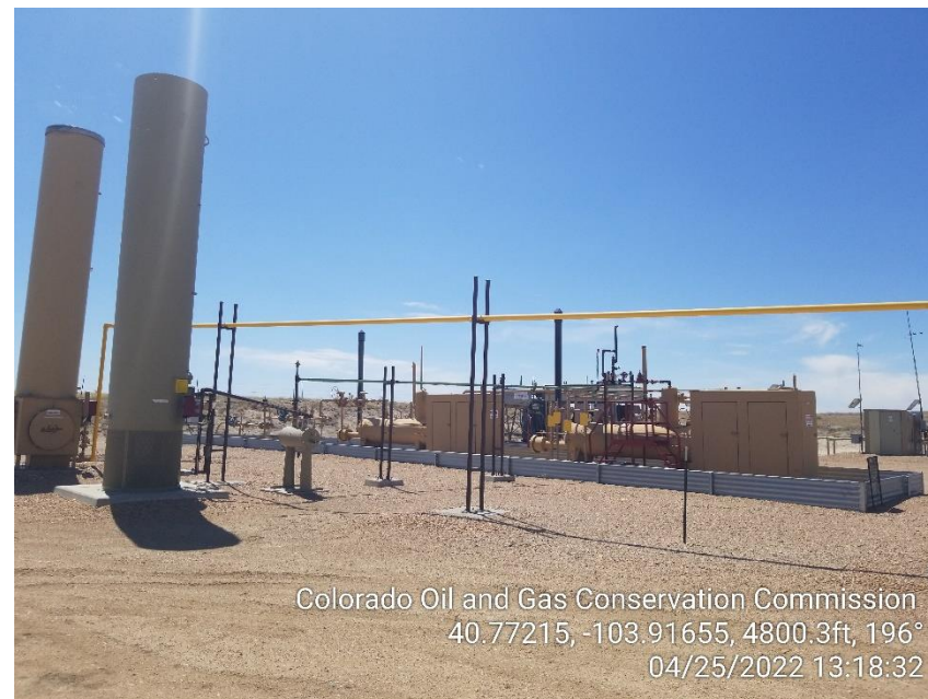
Photo 4 – ECDs and Separators
