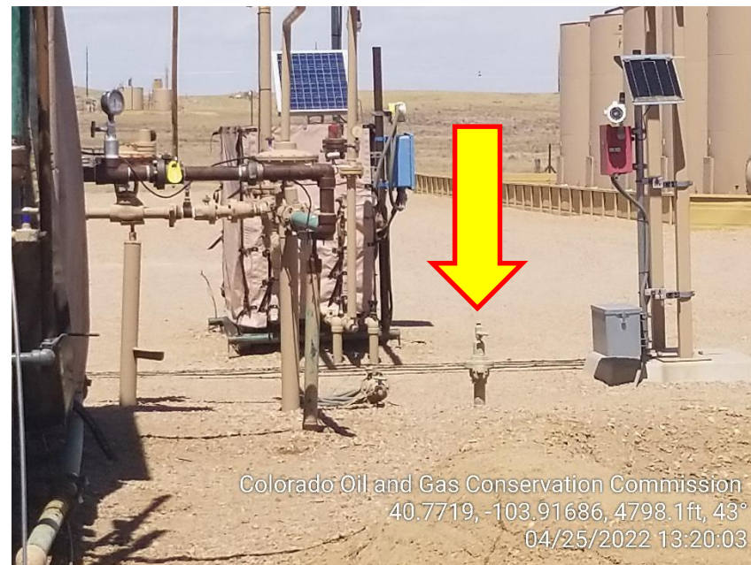
Photo 8 – Unmarked Riser
