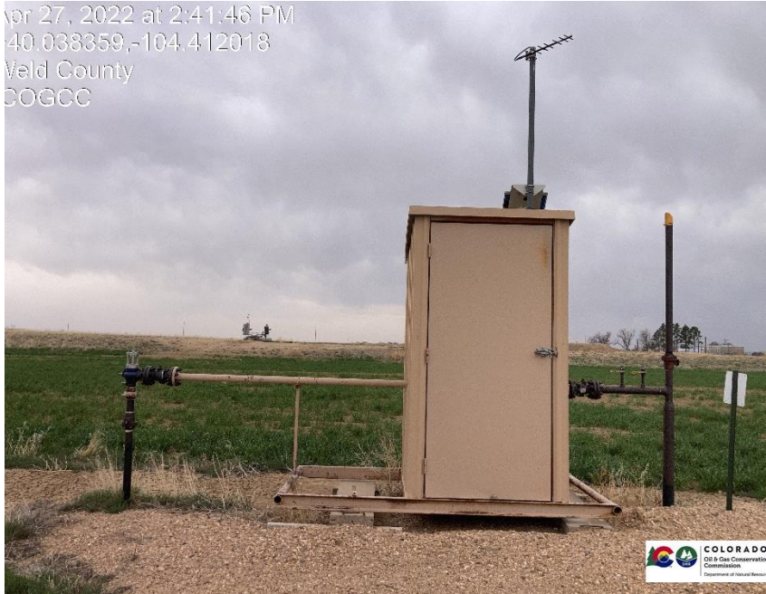
Pic 7 Gas Meter run
