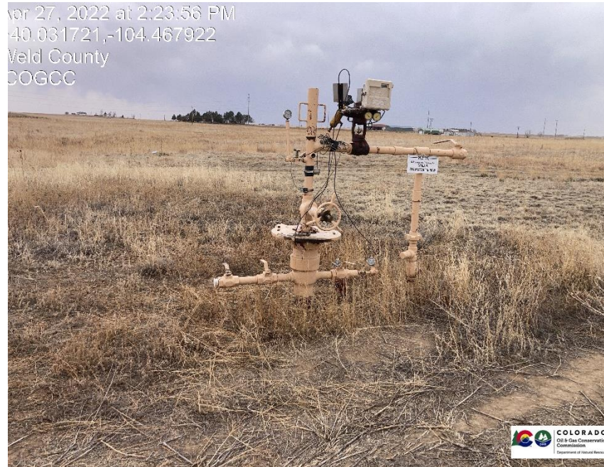
Pic 1 wellhead
