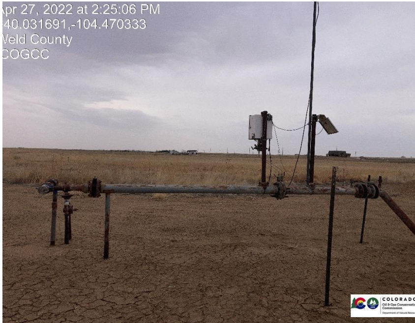
Pic 3 Gas meter run
